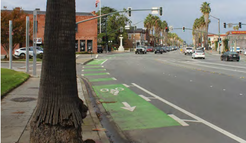
Figure 27: Example of Bike Lane Extension Through Intersection
