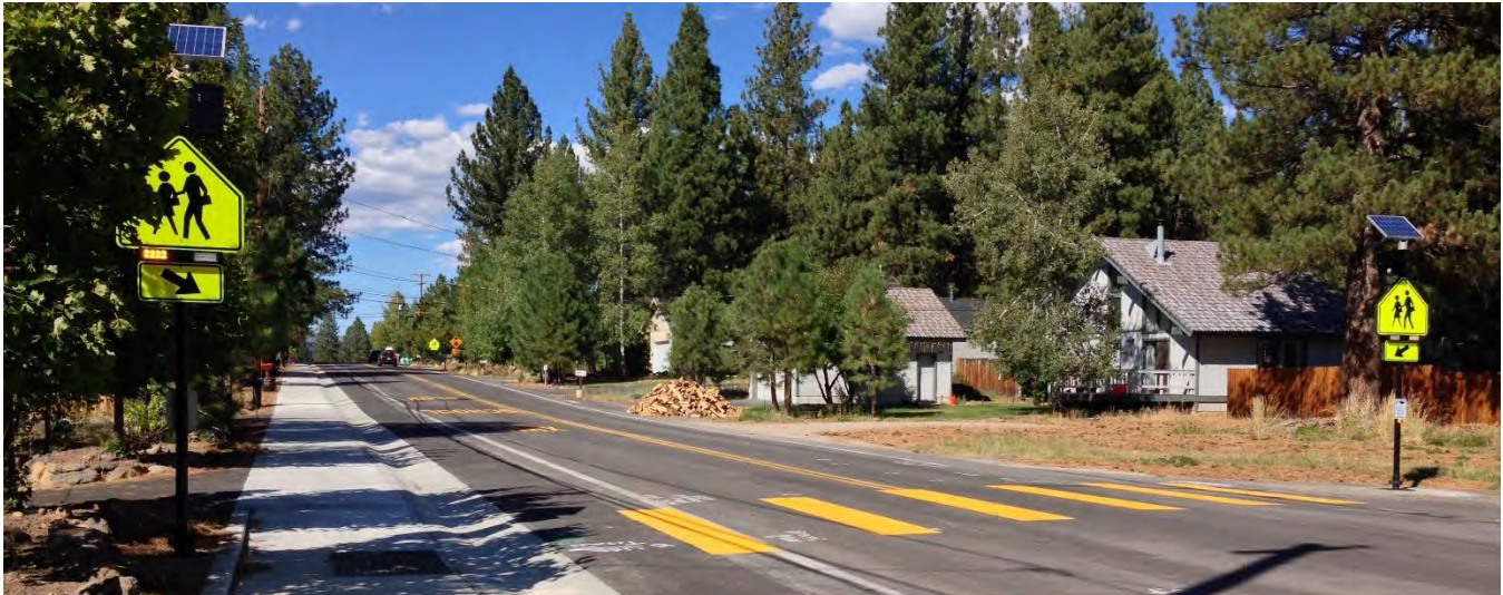
Figure 21: Example of Enhanced Pedestrian Crossing with RRFB
