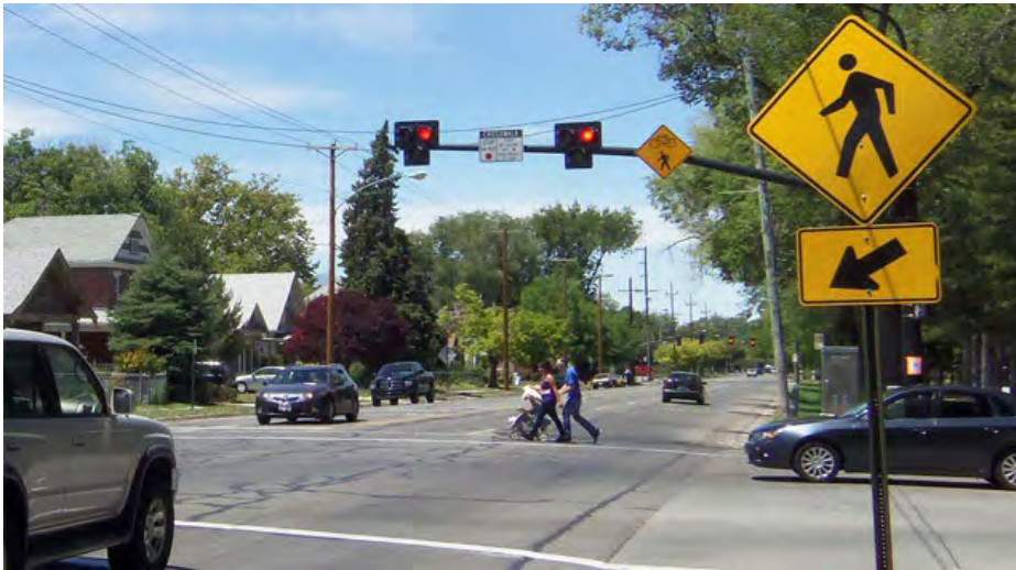
Figure 22: Example of Pedestrian Hybrid Beacon
