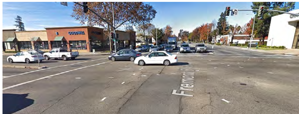
Figure 30: Example of Pavement Markers Delineating Turning Path of Travel
