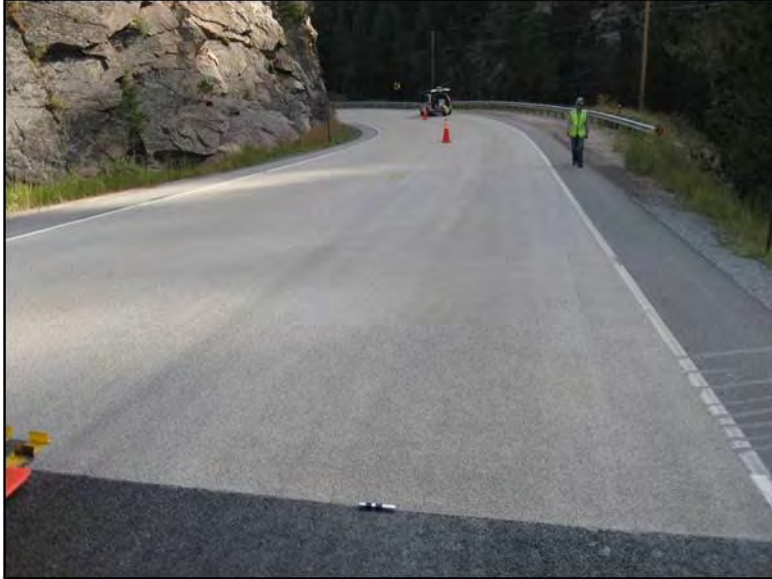
Figure 36: Example High-Friction Surface Treatment Application
