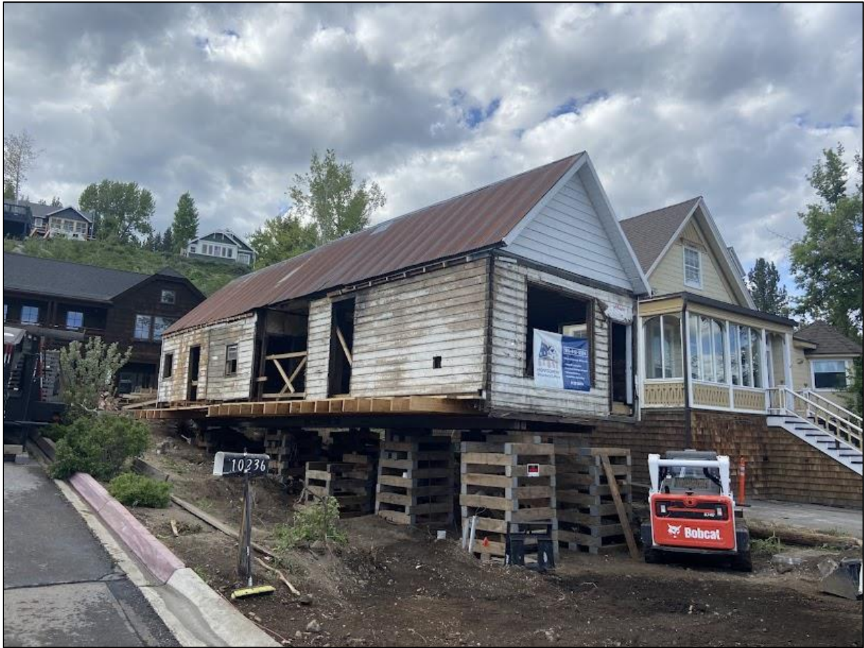
Photograph 6: South (primary) and west elevations of Subject Property during project implementation (showing porch, basement, foundation, front steps, and all windows and doors removed prior to relocation closer to road). Photo taken by applicant team on May 29, 2024.
