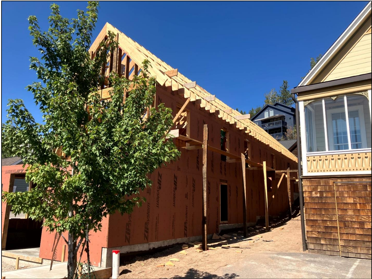
Photograph 8: South (primary) and east elevations of Subject Property during project implementation (showing relocation, all siding, roof materials, windows, and doors removed, and new fenestration pattern). Photo taken by Town Staff on September 5, 2024.
