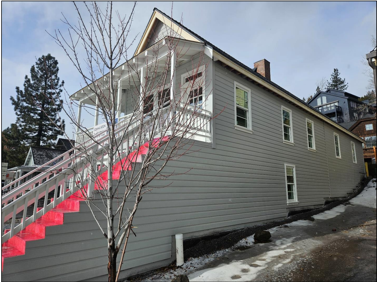
Photograph 12: East elevation of Subject Property near project completion (showing new windows and window arrangement, foundation, and addition marked by siding transition). Photo taken by Broadbent on November 21, 2024.
