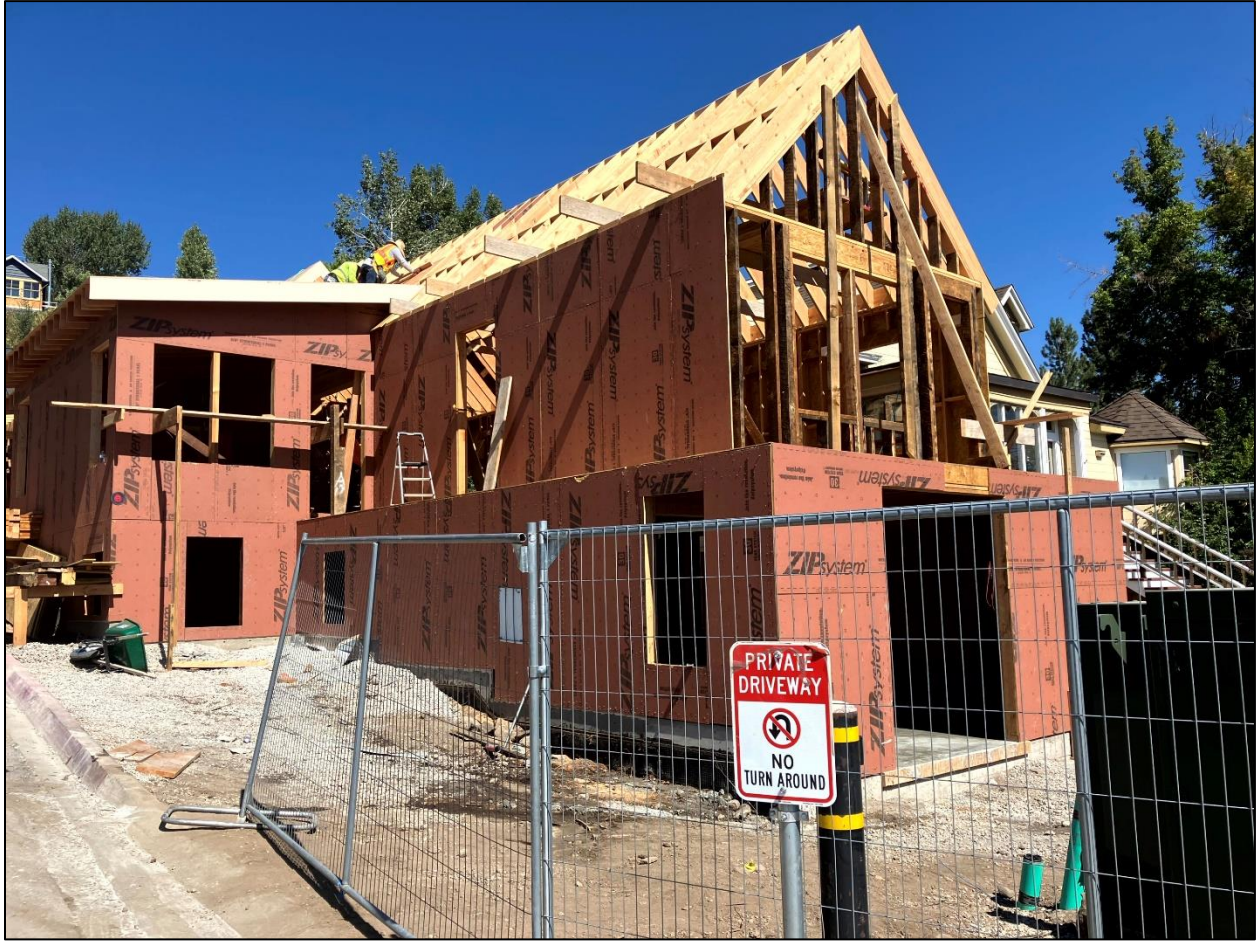
Photograph 7: South (primary) and west elevations of Subject Property during project implementation (showing relocation addition, all siding, roof materials, windows, and doors removed, and new fenestration pattern). Photo taken by Town Staff on September 5, 2024.
