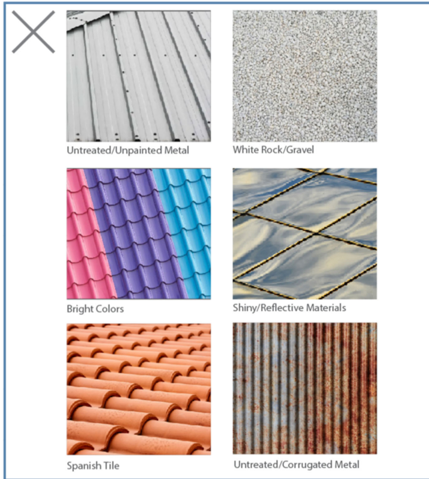
FIGURE 2-X INNAPPROPRIATE MATERIALS ROOF MATERIALS
