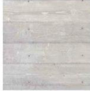
board formed concrete 1x8 board formed
