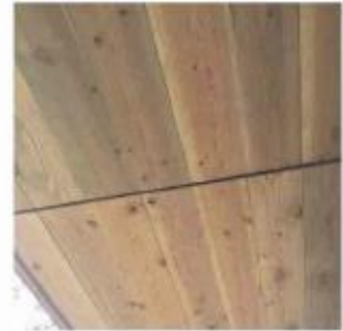
soffits 1x8 1+g grade d doug fir, resawn stain: ginger
