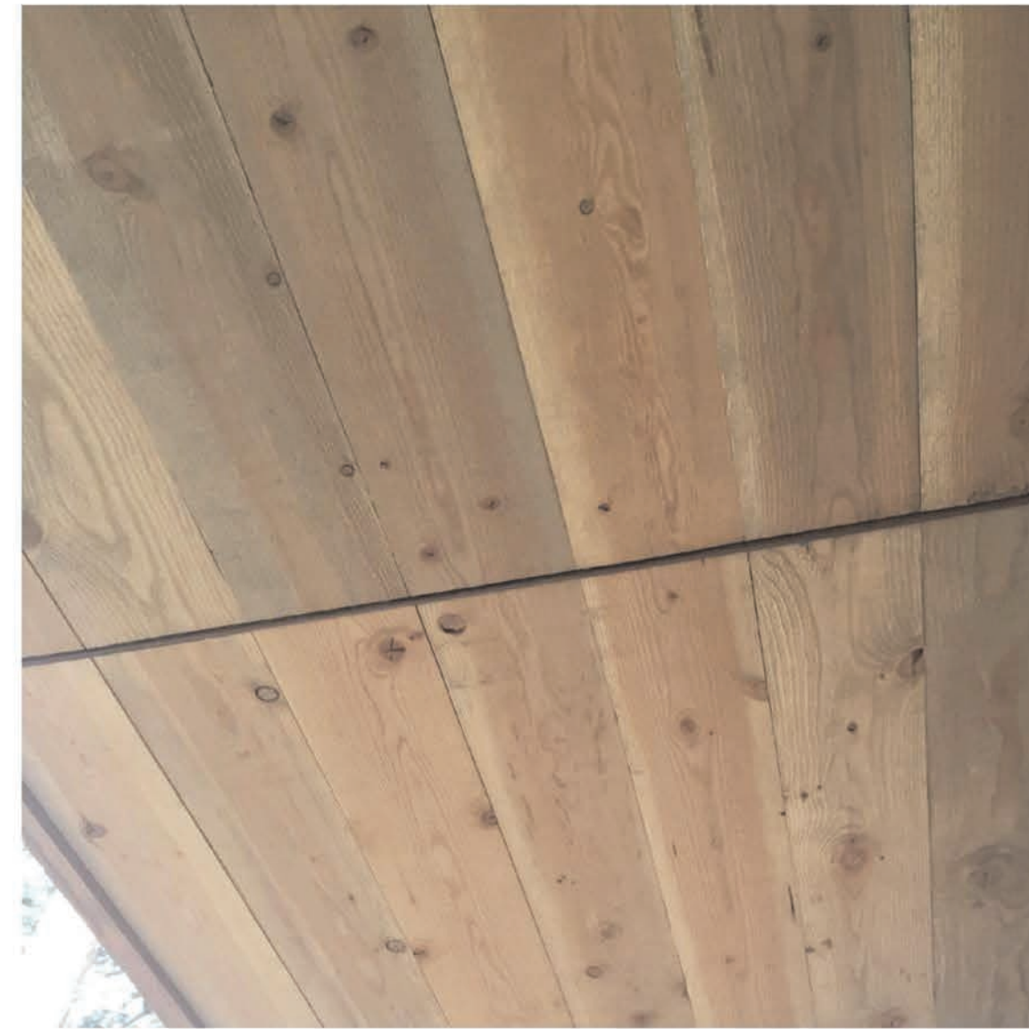
soffits 1x8 t+g grade d doug fir, resawn stain: ginger
