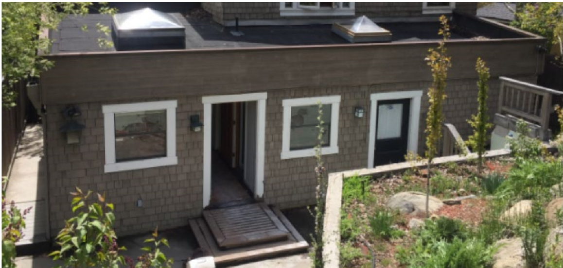
Figure 11 – Existing fenestrations in modern rear (north) addition at ground floor
