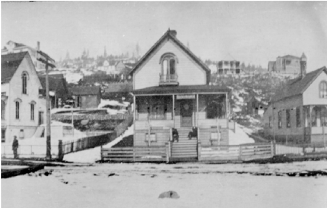
Figure 4 – Historic photo of the property (center) c. 1902-1906
