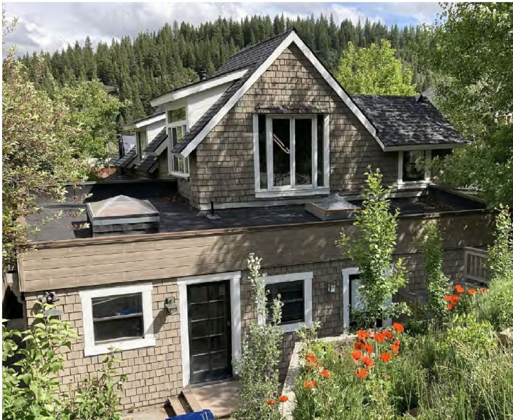
Figure 6 – Existing rear (north) elevation of project site
