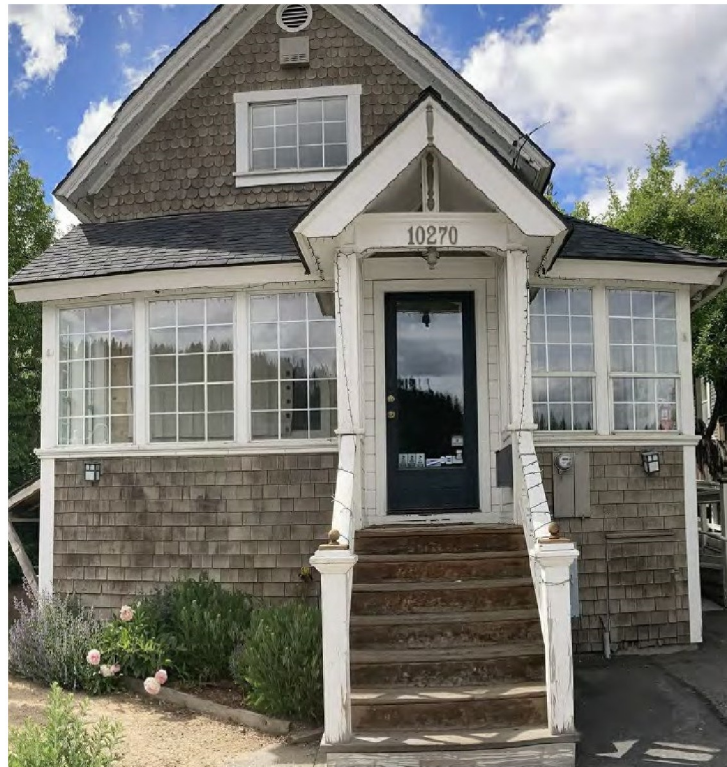
Figure 9 – Existing front porch
