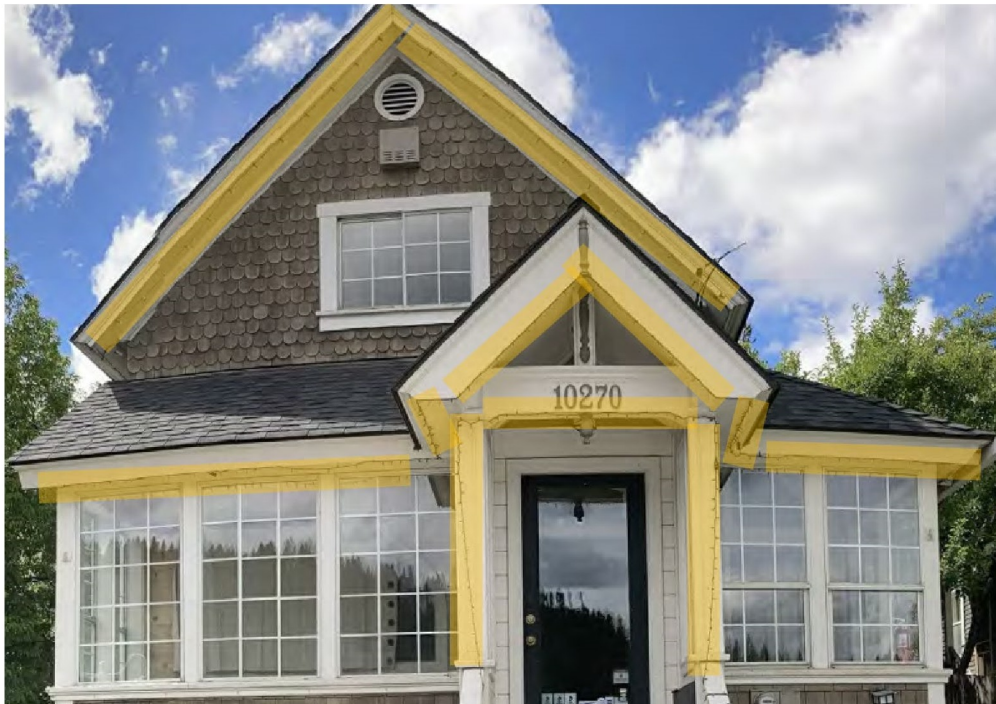
Figure 22 – Existing holiday string lights (highlighted)
