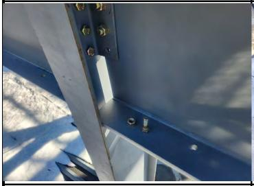
Bolt removed from structure - observed to be in good condition
