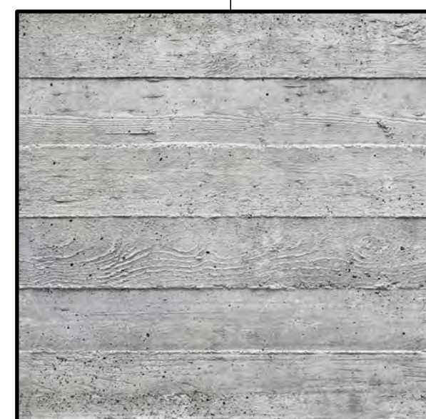
BFC: BOARD FORM CONCRETE AT FOUNDATION AND RETAINING WALLS
