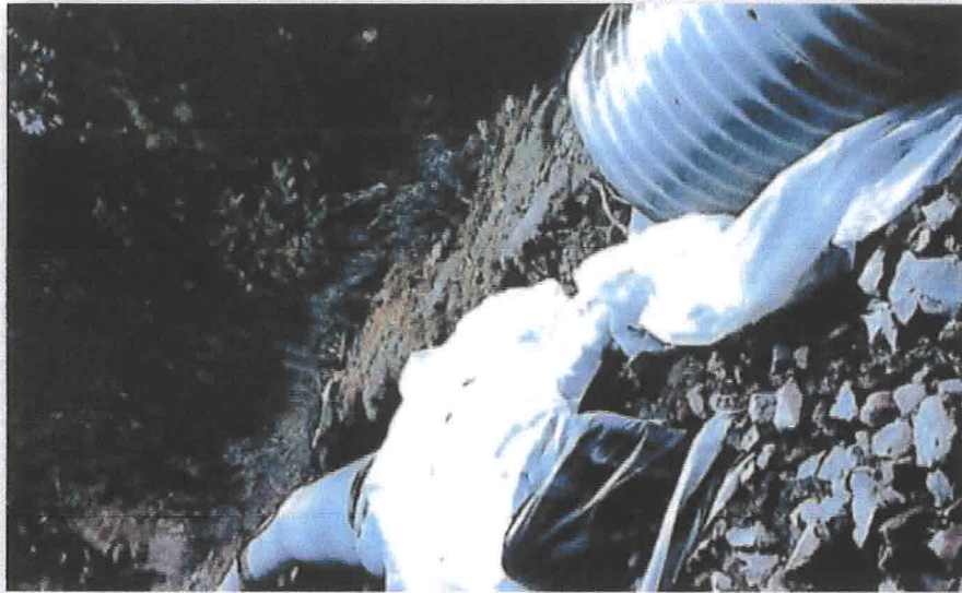
I-80 Drainage Culvert
