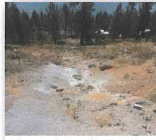
Heavy channelization from I-80, looking downhill.
