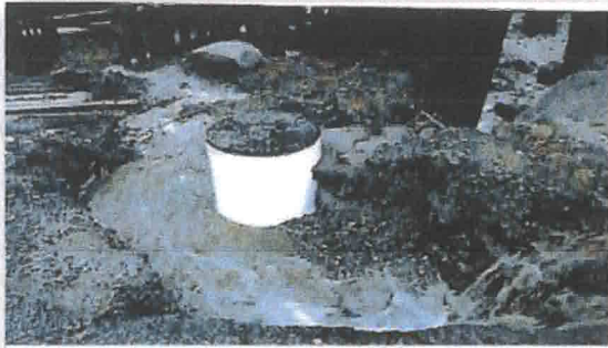
Utility infrastructure on Reed Avenue West
