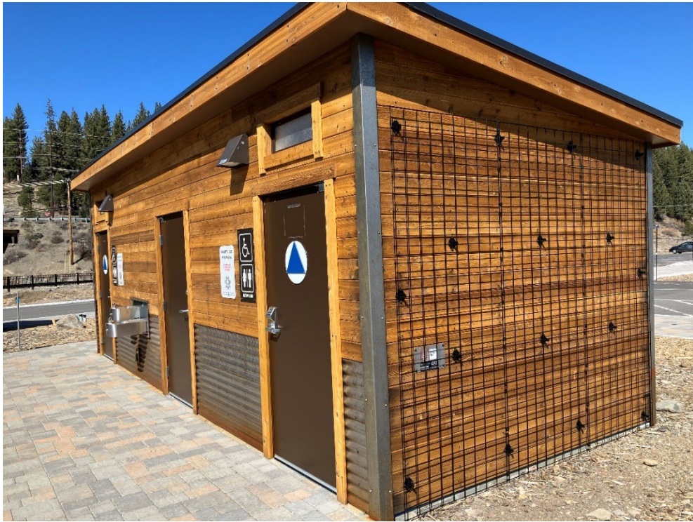
Photo 7: Metal Trellis on the side of the Public Restroom
