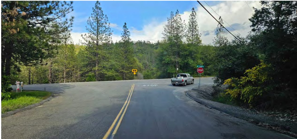
FIGURE 44: OUTINGDALE ROAD ACCESS FACING EAST
