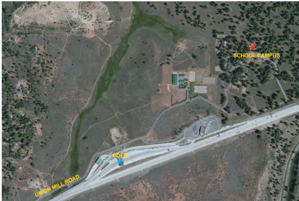
Figure 1: Area Map Showing the Location of the School Campus and CDFA Facility
