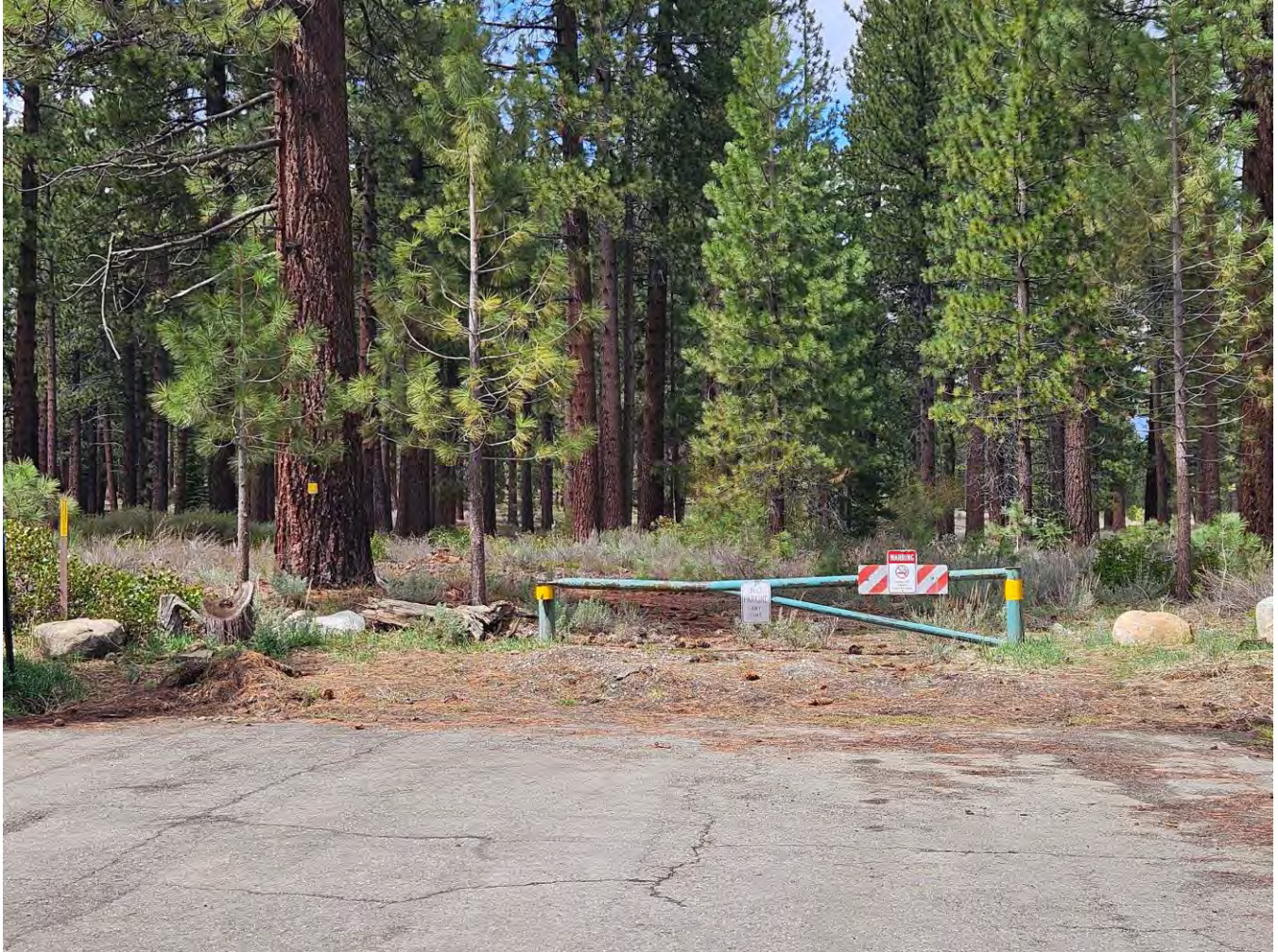
FIGURE 49: GOLDEN BEAR TRAIL EXIT ROAD AT JACARILLO TRAIL ROAD
