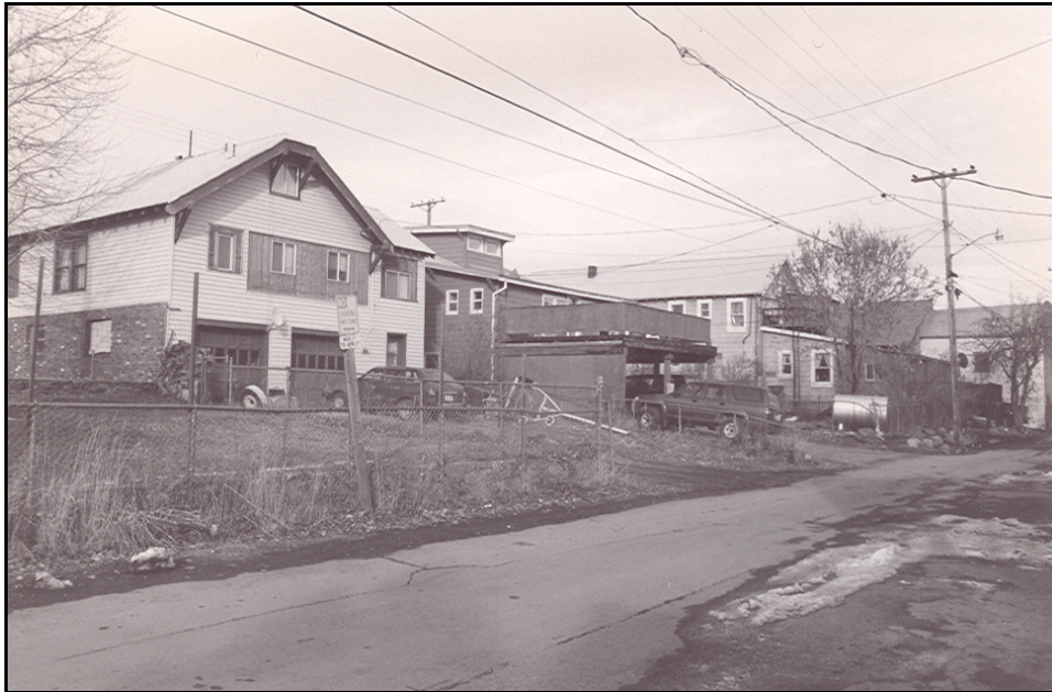
West and south elevations; northeast view from Riverside Drive, 11/20/1998; Acc. #134-15-2. Resource #149 is the dark building at the center (note balcony and carport).
