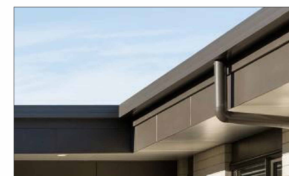
F ROOF FACIA COLOR: CHARCOAL CLASS A FIRE RATED
