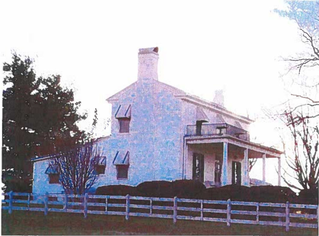
Side view from east
