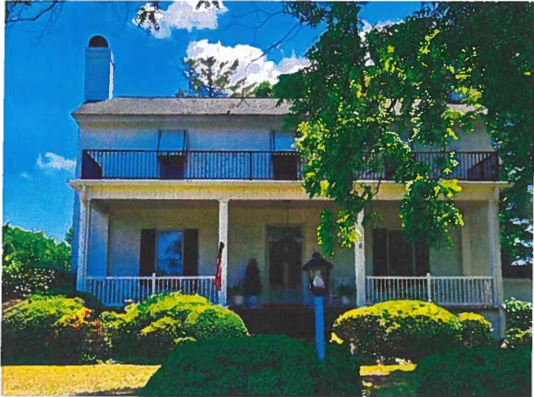
Front view from north
