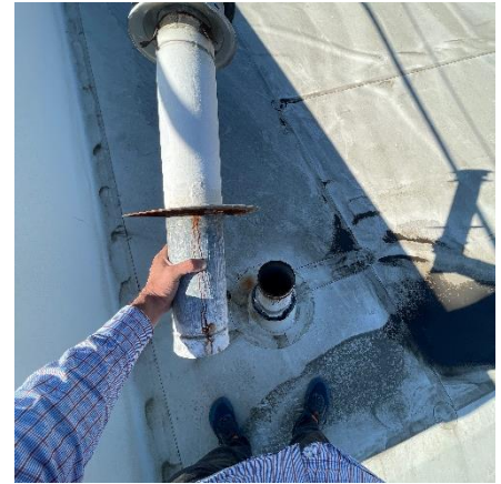
Detached HVAC Vent Assembly
