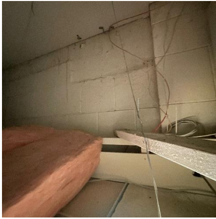
2x4 Stud Wall Adjacent to CMU Block Stud Walls Joined Above Drop Ceiling
