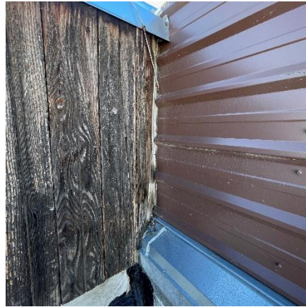
Improper Sealing/Flashings
