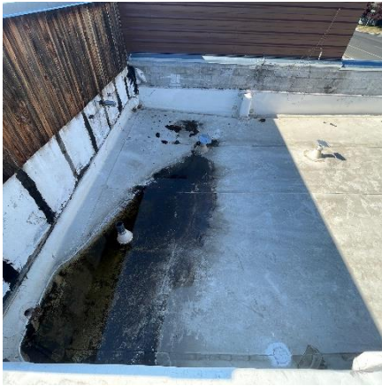
Roof Ponding and Clogged Drain
