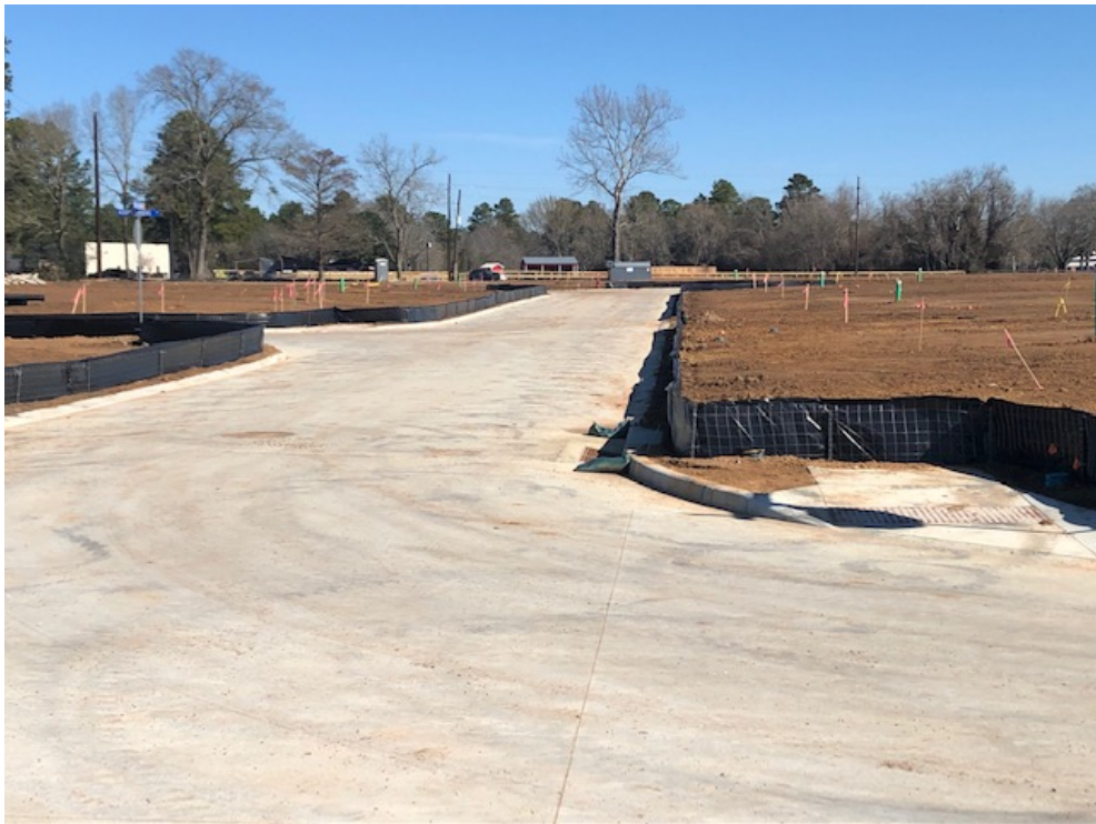
Intersection of Silver Maple Crossing and Wood Leaf Park facing North
