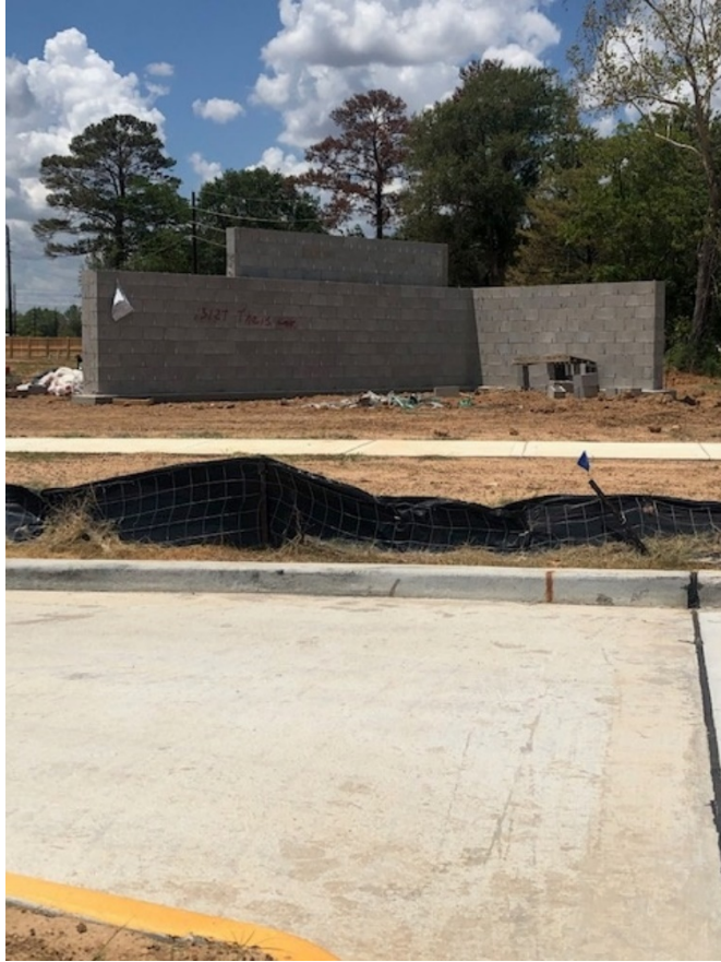
Entry Monument at This Lane (under construction)
