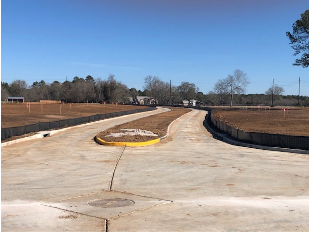
School Street facing North toward This Lane entrance
