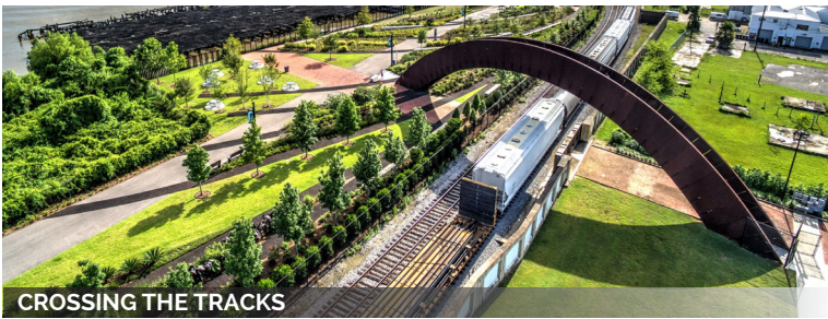
CROSSING THE TRACKS
