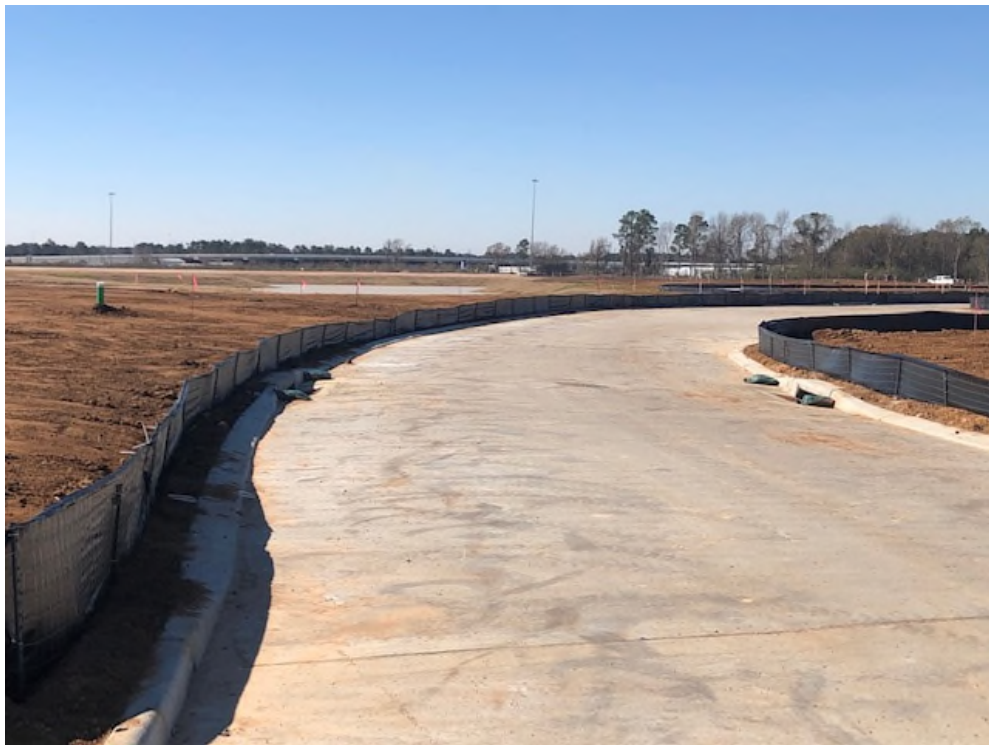
Intersection of Silver Maple Crossing and Wood Leaf Park facing South
