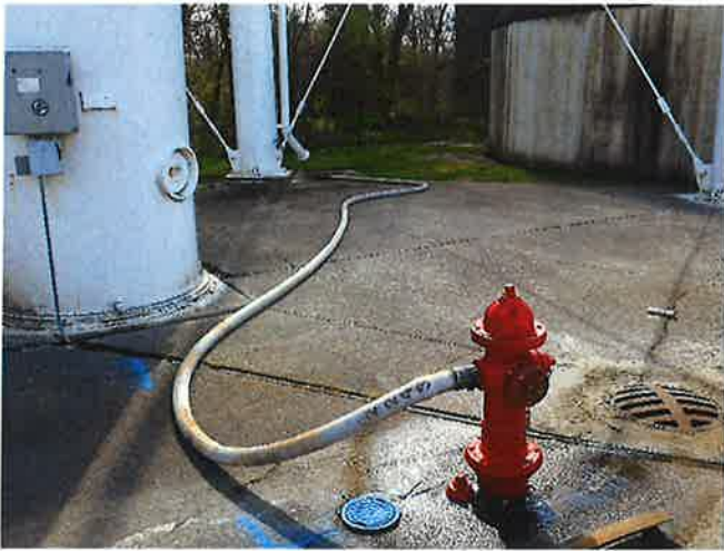
DRAINING OF TOWER IN PROGRESS
