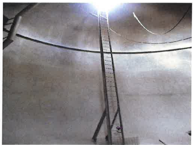
PRIMER COATING IN PROCESS
