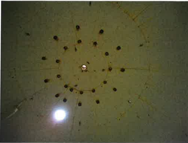
OLD CP PORTS TO BE COVERED WITH WELDED PLATES
