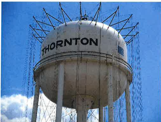
CONTAINMENT SYSTEM INSTALLED
