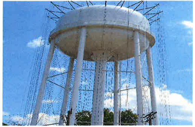
INTERMEDIATE COAT COMPLETED
