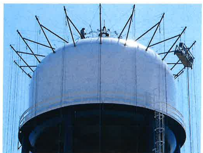
FLOUROPOLYMER TOPCOAT IN PROCESS
