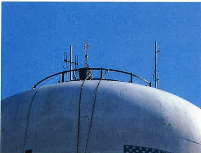
NEW ROOF CORRAL INSTALLATION
