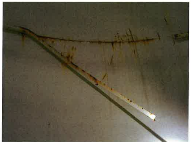
STIFFENER RING CORRODED AND DETACHED FROM TANK
