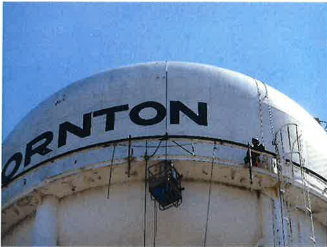
CATWALK RAIL EXTENSION IN PROCESS
