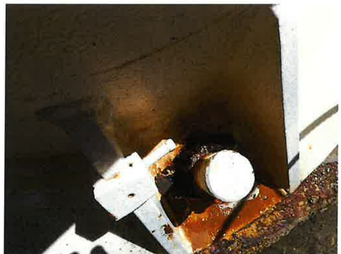
GENERAL CORROSION W/UNDERCUTTING
