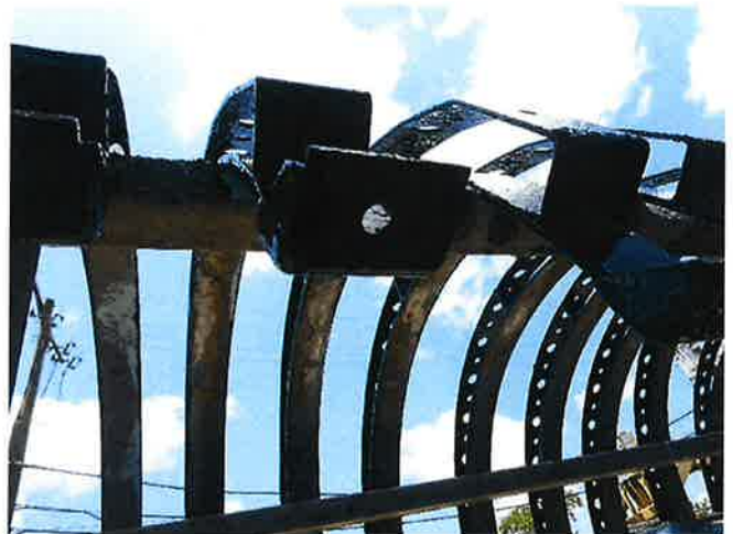
METAL BANDS CLEANED AND COATED
