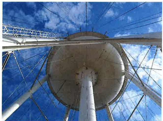
TANK EXTERIOR WATERJET CLEANED
