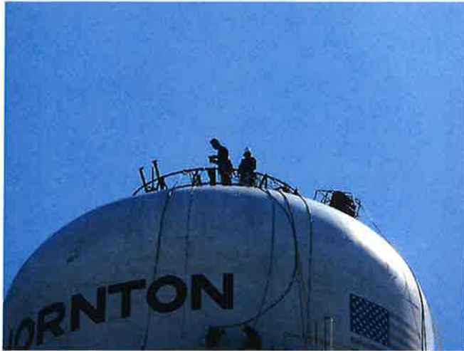
ROOF CORRAL FABRICATION IN PROCESS
