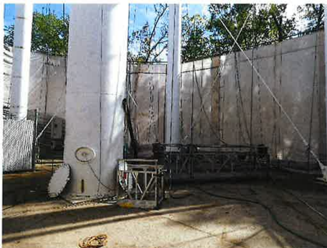
TANK EXTERIOR WATERJET CLEANED
