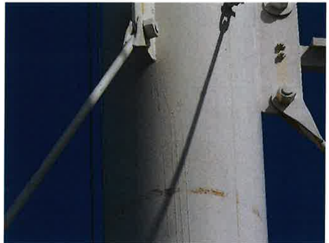
RUNS IN COATING PREVIOUS APPLICATION
