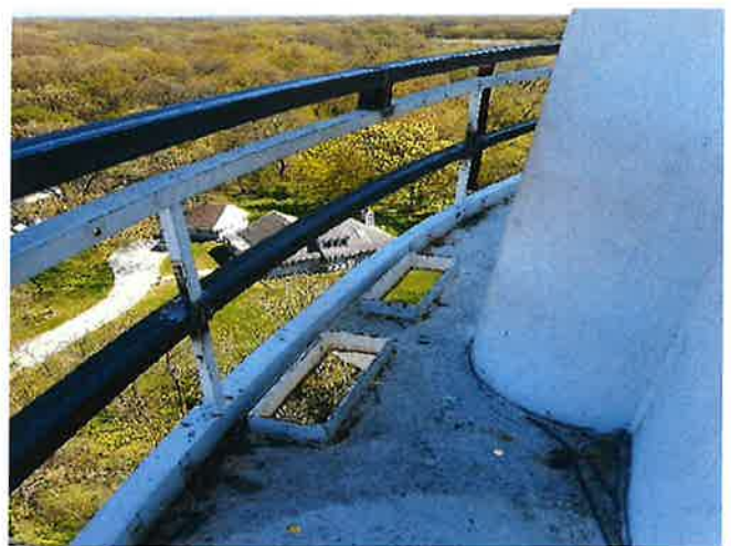
CATWALK HANDRAIL RAISED TO 42"
