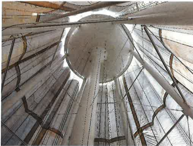
INTERMEDIATE COATING IN PROCESS
