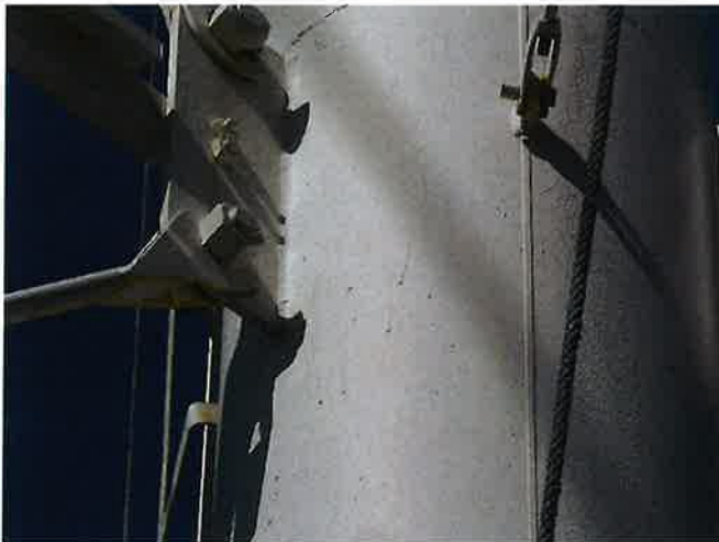
RUNS IN COATING PREVIOUS APPLICATION
