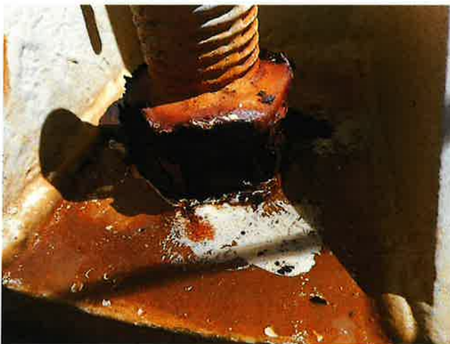
GENERAL CORROSION W/UNDERCUTTING
