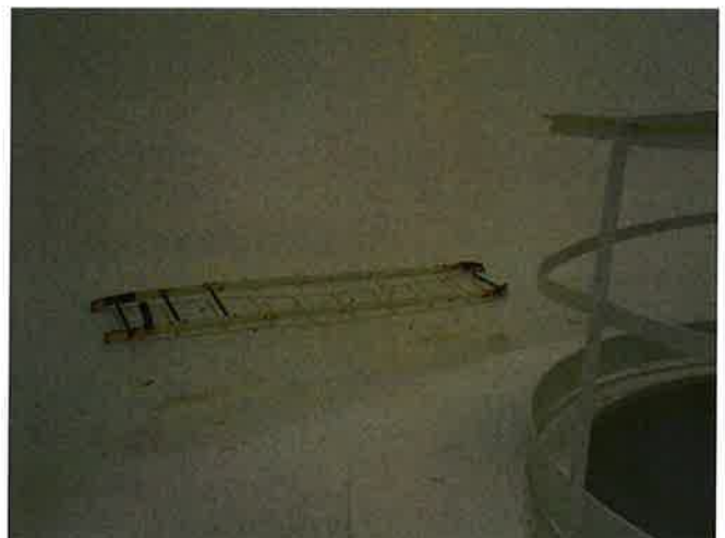
WET INTERIOR LADDER CORRODED AND DETACHED FROM WALL
