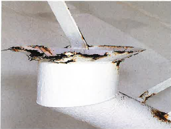
TOP OF OVERFLOW PIPE CORROSION
