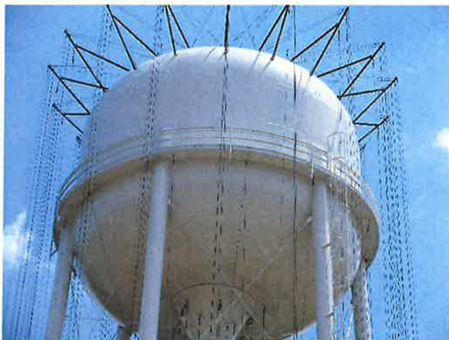
INTERMEDIATE COATING IN PROCESS
