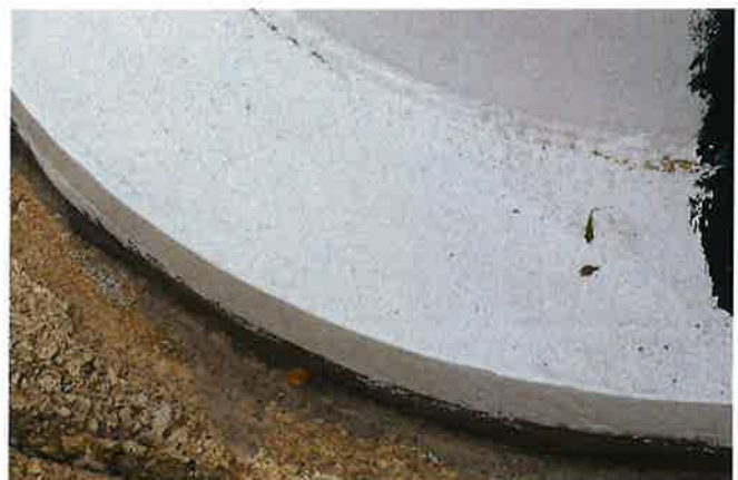
CONCRETE AREAS AROUND BASES HAVE BEEN REPAIRED/COATED
