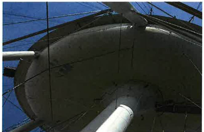
SPOT SANDBLASTED AREAS OF CORROSION ON TANK EXTERIOR
