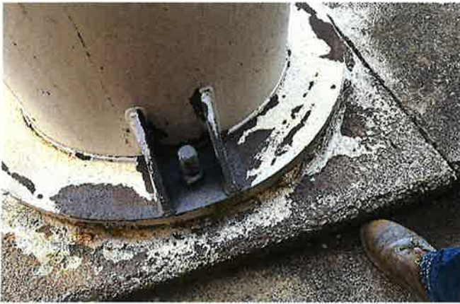
SANDBLASTED CORROSION ON/AROUND ANCHOR BOLTS
