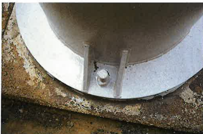
ANCHOR BOLTS AFTER SANDBLASTING
