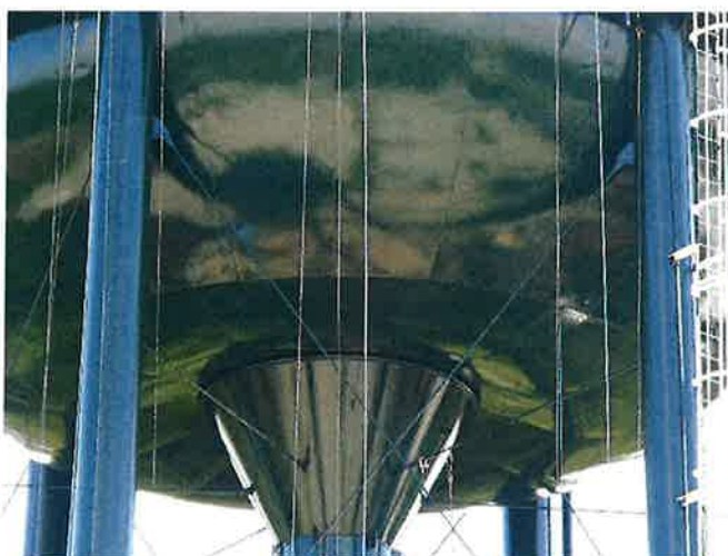
FLOUROPOLYMER TOPCOAT IN PROCESS
