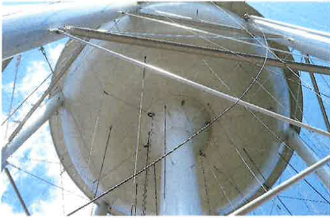
INTERMEDIATE COAT COMPLETED
