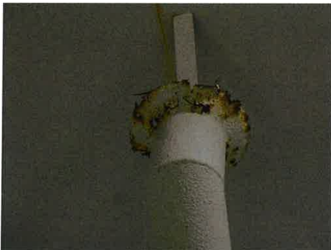
OVERFLOW TOP HAT EXCESSIVE CORROSION
