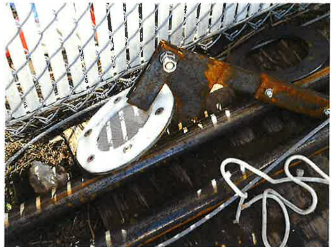
NEW OVERFLOW FLAP GATE
