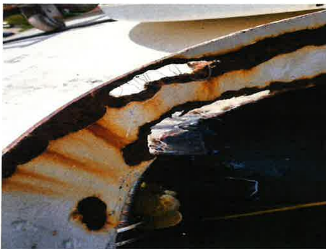
ROOF PLATE AND COLLAR SEVERELY CORRODED
