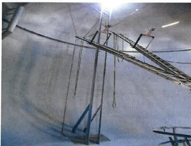
PRIMER COATING IN PROCESS
