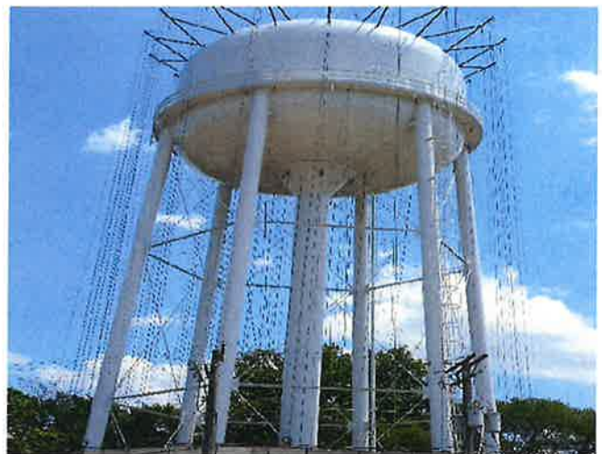
INTERMEDIATE COATING IN PROCESS
