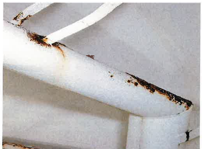
OVERFLOW PIPE CORROSION
