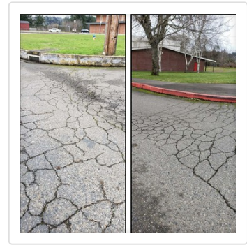
Parking Lot Repairs
