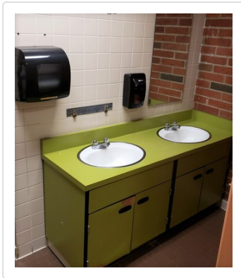
Restroom Repairs & Upgrades
