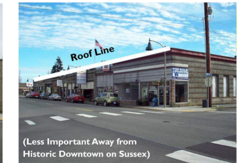
Similar Roof Lines
