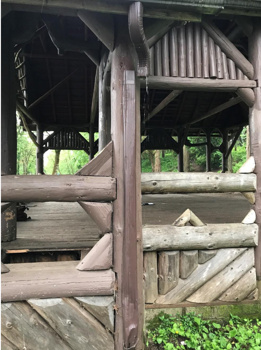
Picture 11 – damaged downspout
