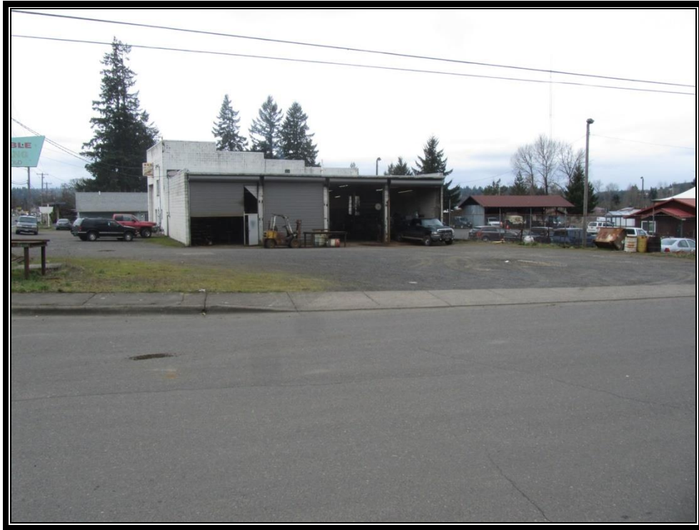
View of Hutchins/Reliable property from 24 th Avenue frontage. (A12-494)
