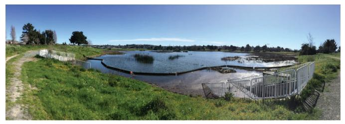
West Yost prepared the detailed design and specifications for the Vallejo Flood and Wastewater District's Lake Dalwigk Detention Basin Improvements project, which included enlarging the lake and designing 2,600 feet of 96-inch bypass pipeline through a congested industrial area.
