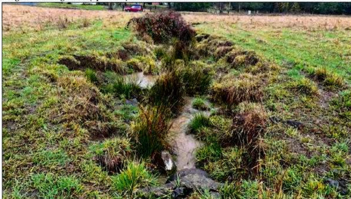
Image 7- Looking south (upstream) at Ditch E and culvert.
