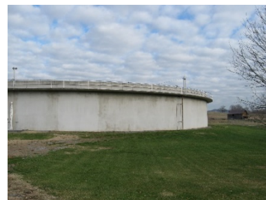
Sludge basin at Bristol, Tenn./Va.
