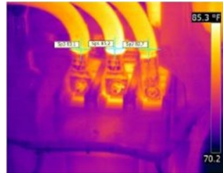
As part of our predictive maintenance program, we will take thermographic images of all newly installed equipment to identify construction issues and maintain this practice ensuring extended lifecycle for all equipment.
