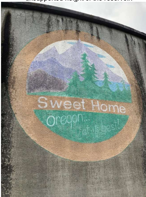
Figure 6.12 49 th Avenue Reservoir 2.0M Wall
