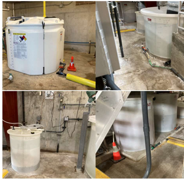
Figure 6.3.4 Tanks without Restraints
