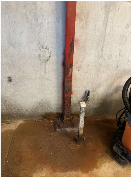
Figure 6.3.3 Corrosion at Steel Columns
