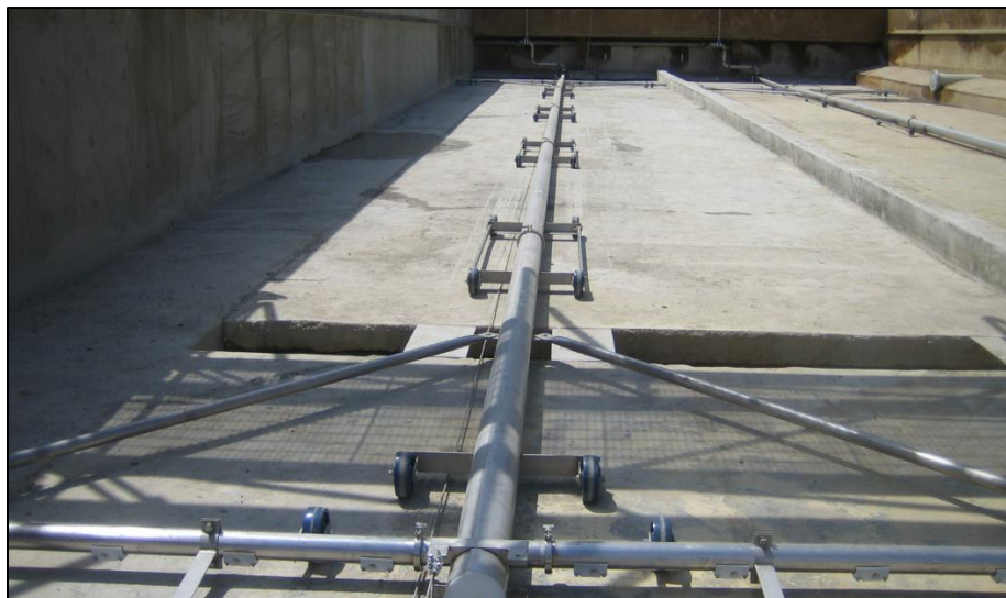
Figure 7-5. Meurer Research Hoseless Vacuum Sludge Collector
