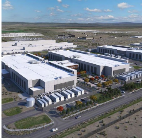
Aerial view of the Meta data center campus in Prineville.
