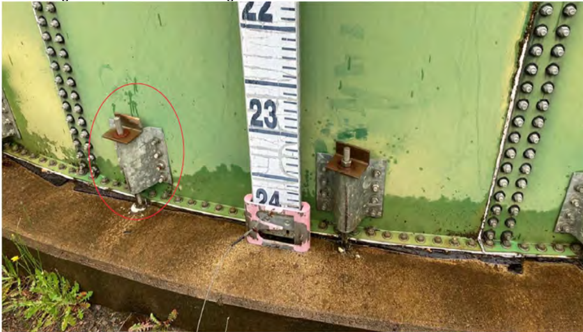
Figure 6.7 Strawberry Reservoir Anchor Bolts
