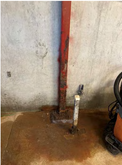
Figure 6.3.3 Corrosion at Steel Columns Figure 6.3.4 Tanks without Restraints
