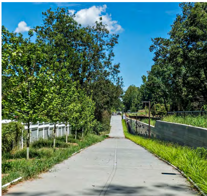
A multi-use path in the vegetated buffer along employment areas could provide easy connectivity from the NSHA to Foster Reservoir and into town.
