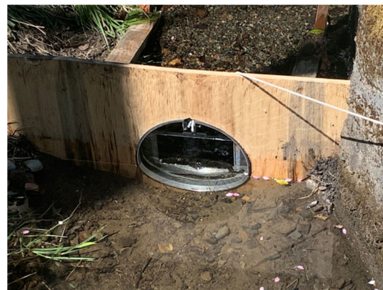
Flow Level After Repair
