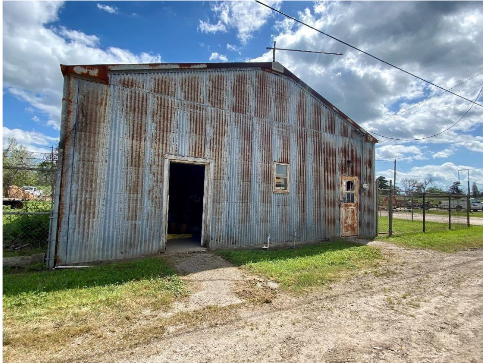
North side of building
