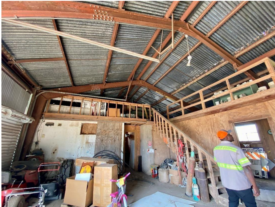
Steel beams inside building
