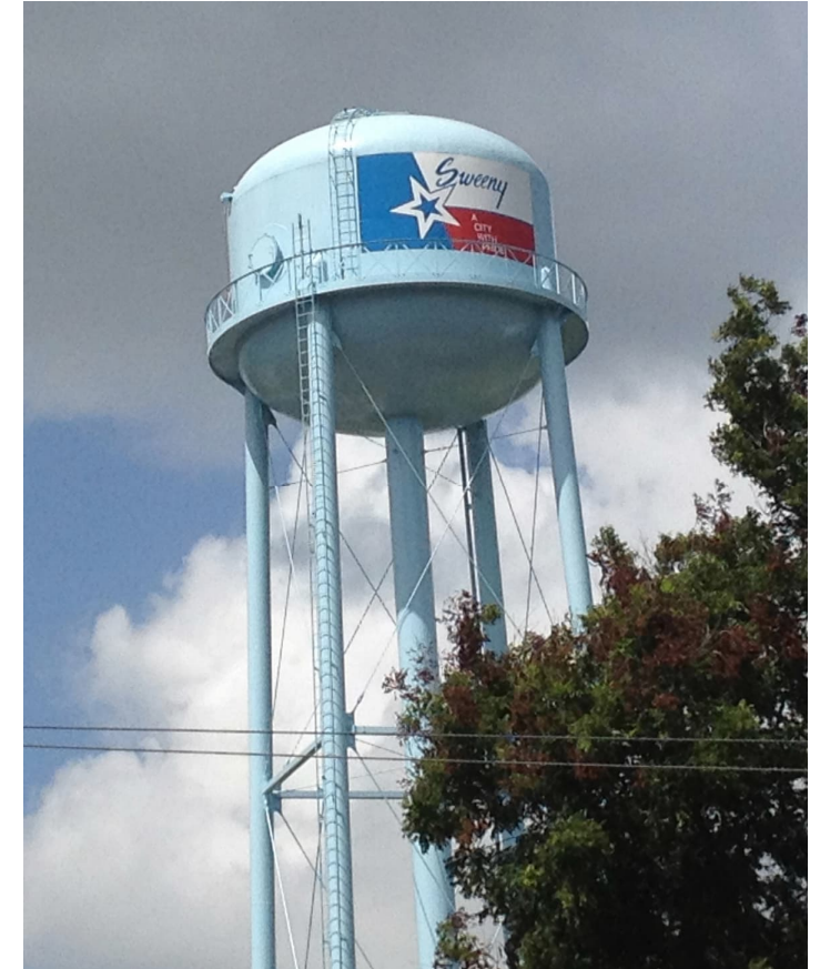
Peach Street elevated storage tank
