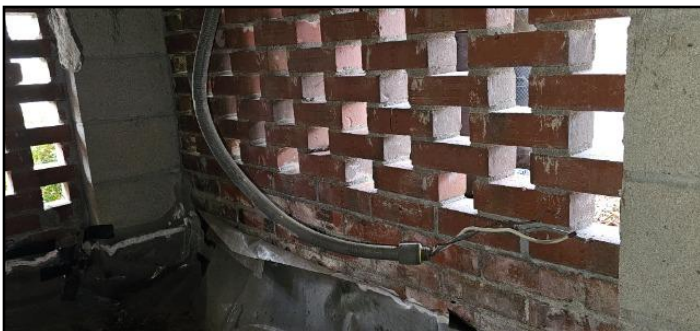
70. Crawlspace below grade
