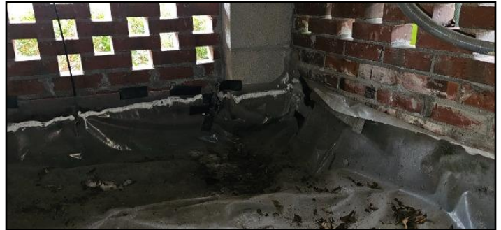
69. Crawlspace below grade
