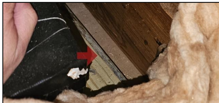
46. Edge of drywall visible from the attic
