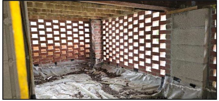
55. Crawlspace below grade
