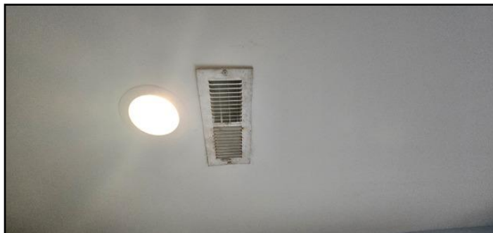
24. Visible growth on register
