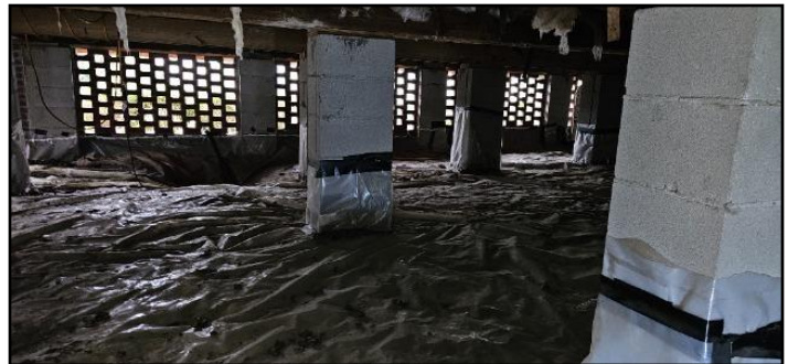
53. Vapor barrier on crawlspace floor
