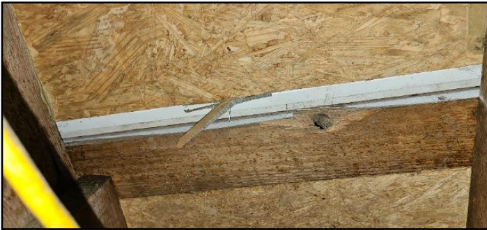
56. Drywall form middle wall visible
