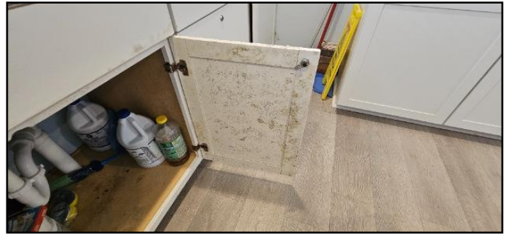
26. Visible growth on cabinets
