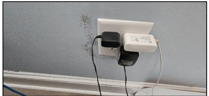
8. Visible growth around outlet
