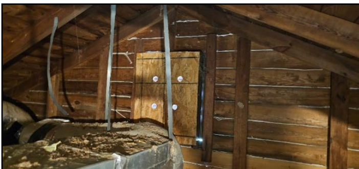
37. Gable vent covered with plywood
