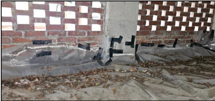
68. Vapor barrier "taped" to wall
