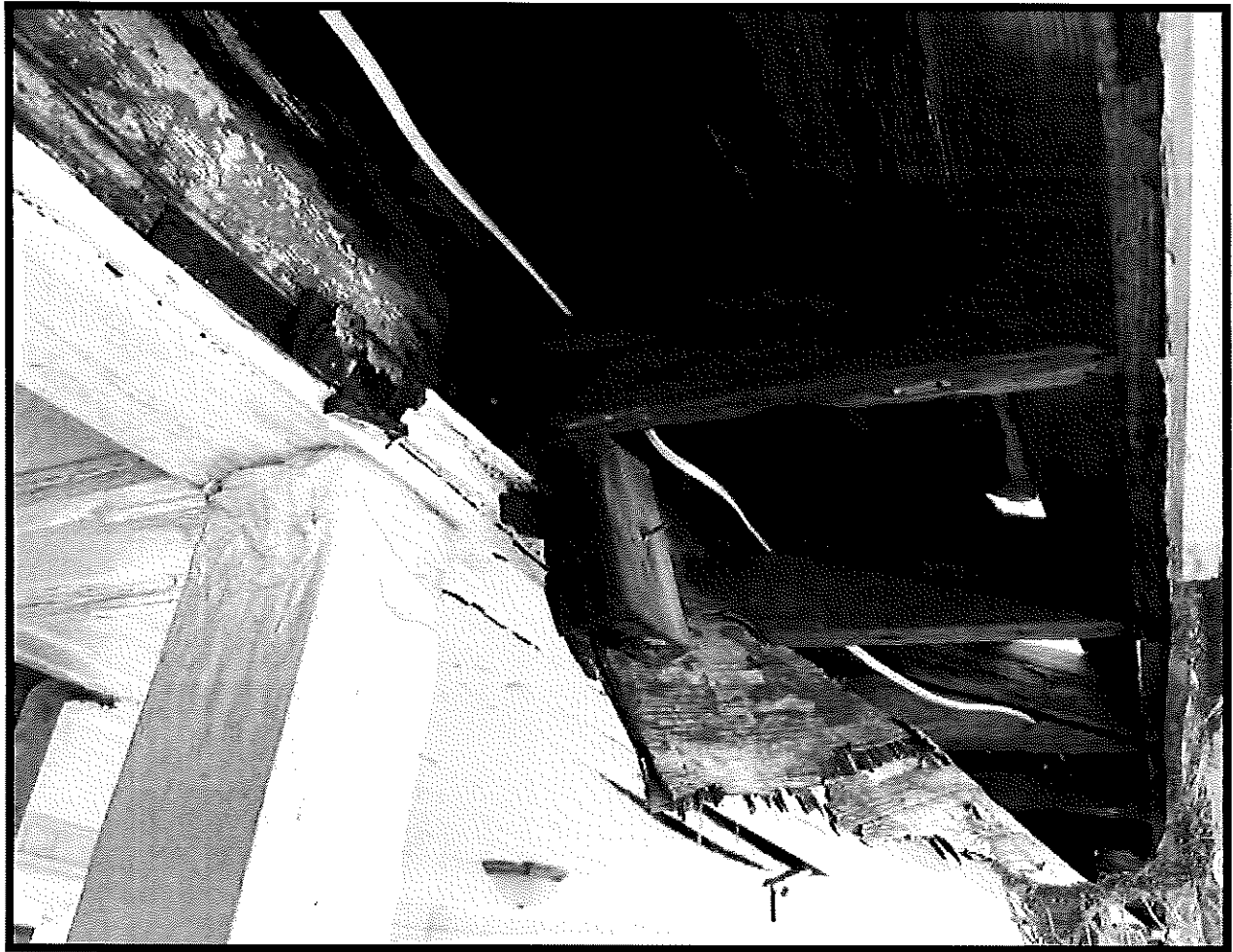
Photo #1: Significant water damage was observed to the roof system associated with the front porch/carport structure.
