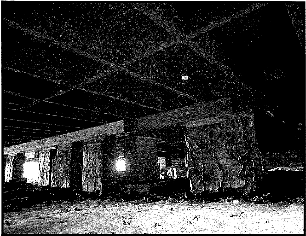
Photo #8: The floor system is comprised of new/treated components. New girders are present which are supported upon some residual dry-stacked block piers. No floor insulation is present.
