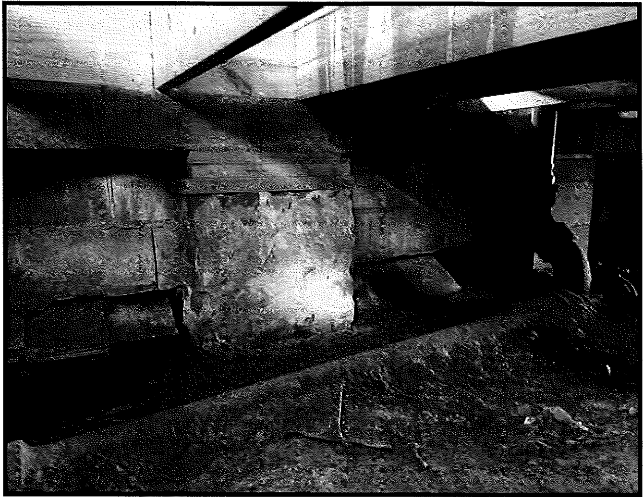
Photo #6: The masonry front porch perimeter exhibits damage to its interior perimeter, as noted from the crawlspace.
