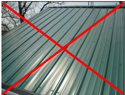
3.1.4 Inaccurate Metal Roof Example
