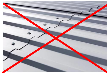
3.1.5 Inaccurate Metal Roof Example
