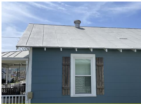
3.1.1 Original Terne Roof
