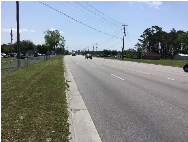
NC 24 (Corbett Ave) looking east away from Queens Creek Rd & Middle School Exit.
