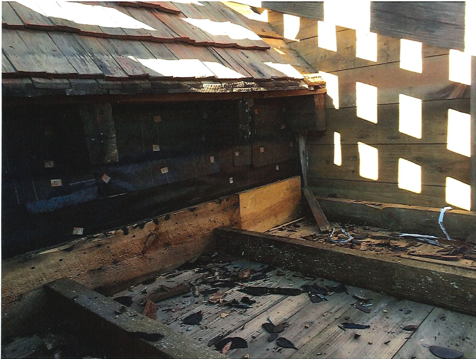
View under porch roof's tie to main roof (looking to side facing Main Street) with original framing and original cedar shake shingles
