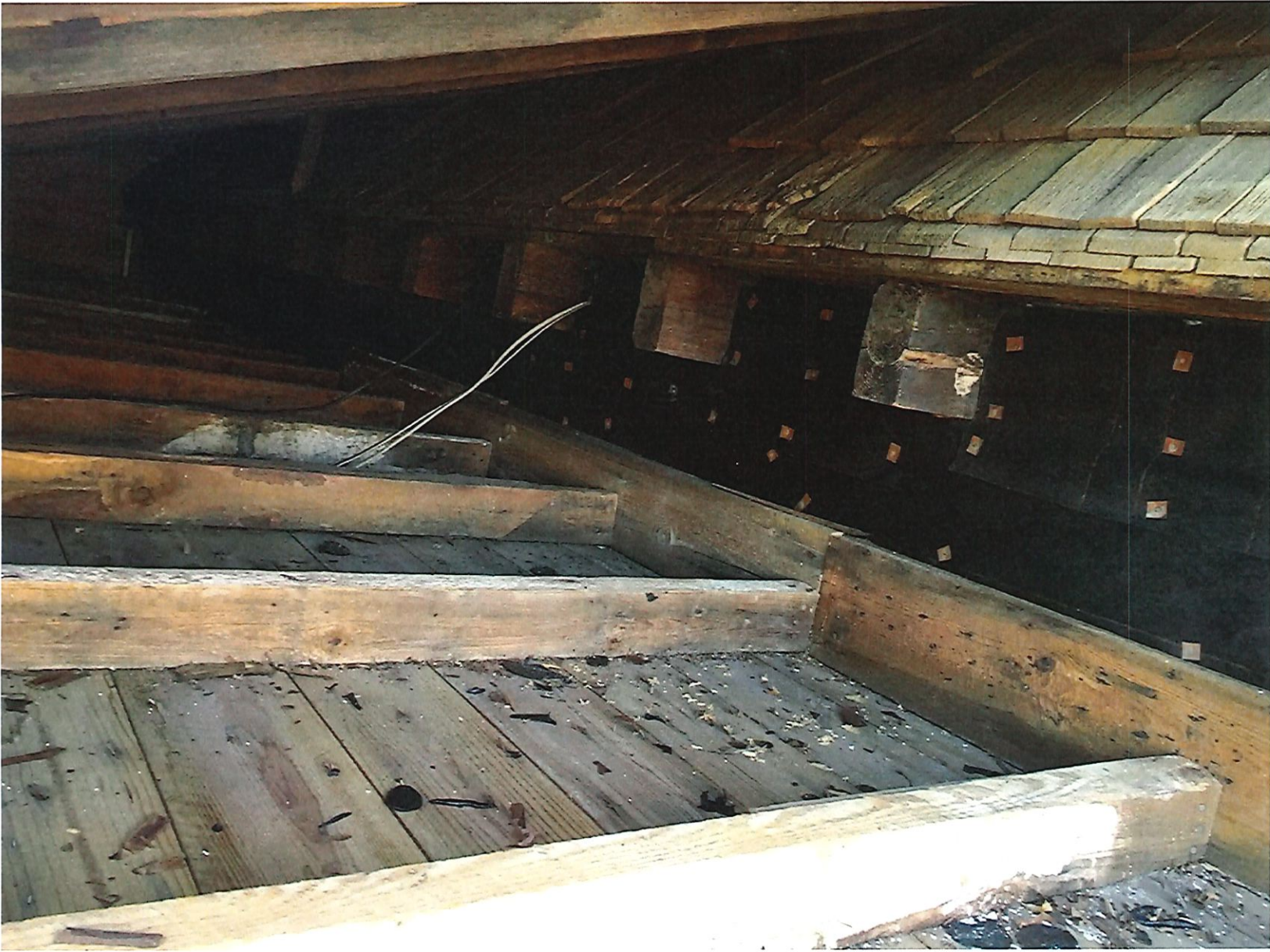
View under porch roof's tie to main roof with original framing and original cedar shake shingles
