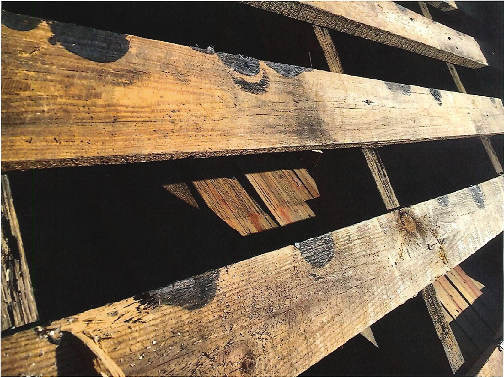
View of Top of Porch Roof Sheathing with original cedar shake shingles underneath on portion of main roof
