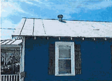
Figure 3.1.1 Original Terne Roof
