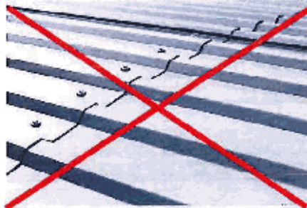
Figure 3.1.5 Inaccurate Metal Roof Example
