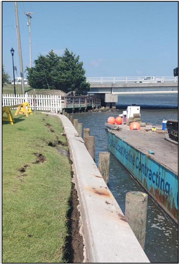
11 pilings added to temporarily hold bulkhead
