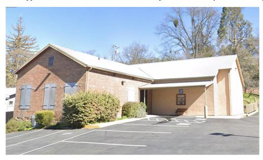
Based on multiple structural assessments (2023), the 1870 unreinforced masonry (URM) portion of the building has severe structural deficiencies and does not meet the Life Safety Performance Level (S-3) of ASCE 41-17, which is necessary for buildings in high seismic areas. A summary of the structural assessments:
