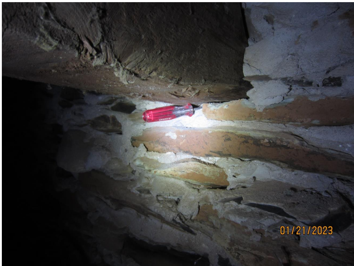
Pic 22 – Stacked shale foundation wall at floor girder at Gridline A
