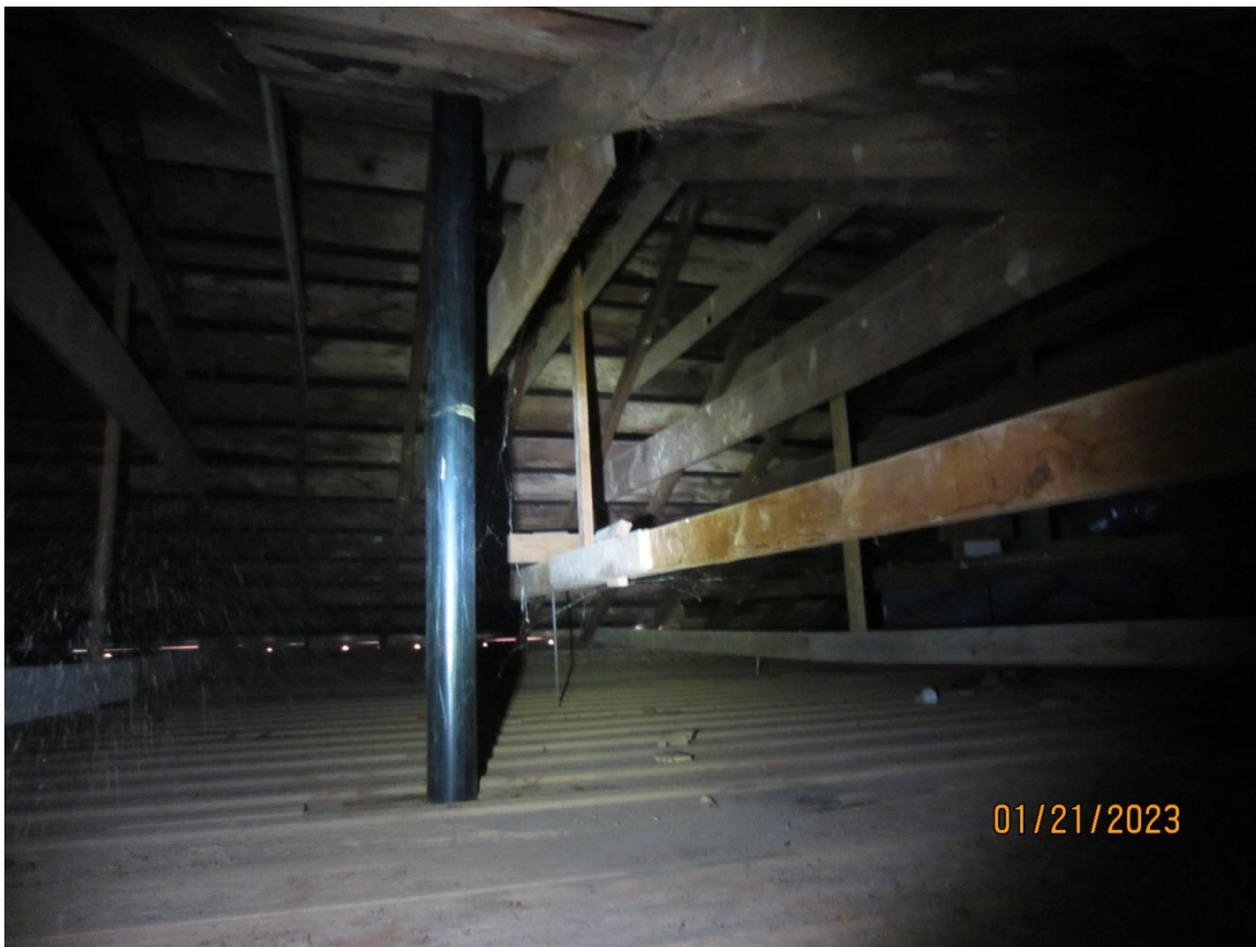
Pic 4 – Collar ties are varying elevations at roof rafters
