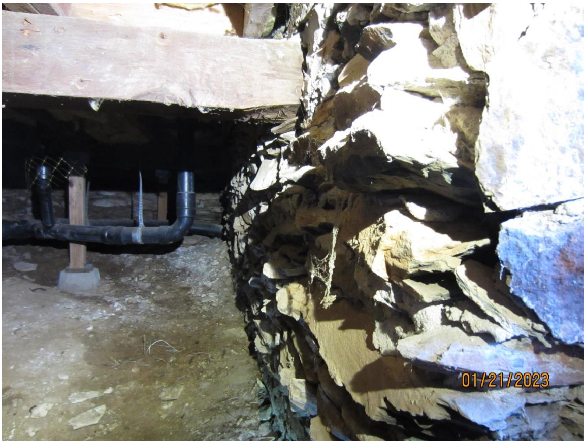
Pic 23 – Stacked shale foundation wall at Gridline A.
