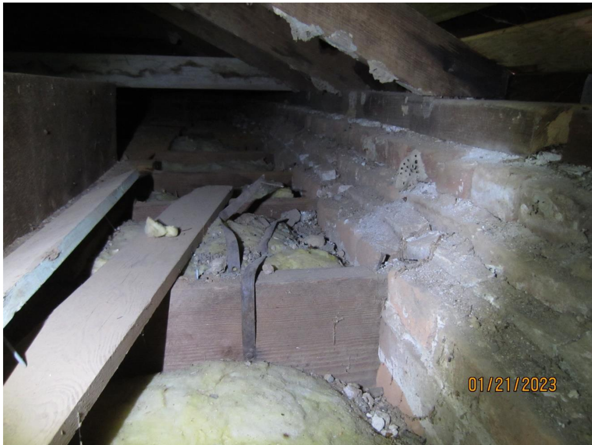
Pic 10 – Attic floor joists built into masonry wall with 1x floor boards removed. Roof rafters on top of wall
