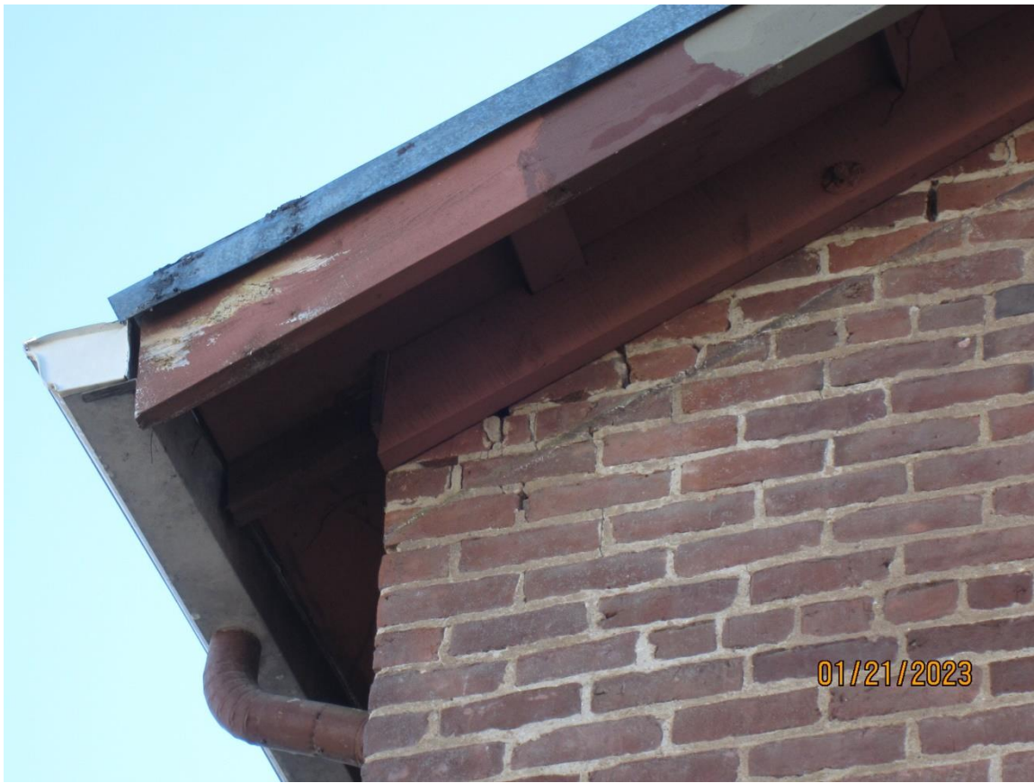
Pic 19 – Loose bricks at top of wall support on north end of west wall
