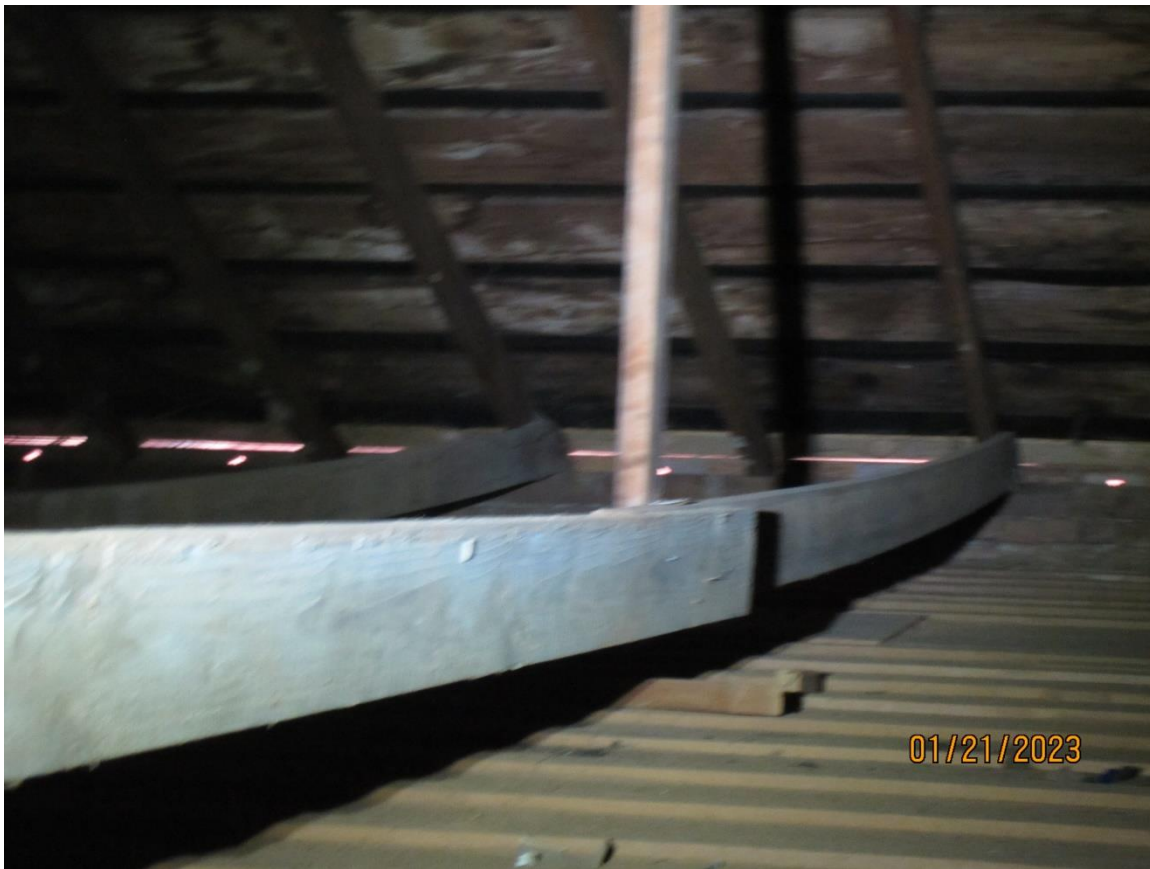
Pic 3 – Sagging collar tie at roof rafters. King Post added at mid-span
