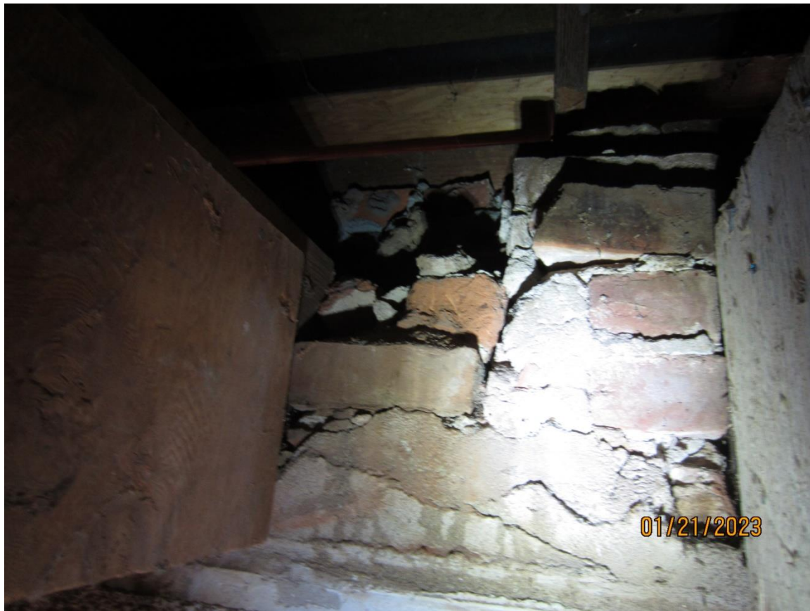
Pic 15 – Loose bricks and weak mortar at attic floor joist repair location
