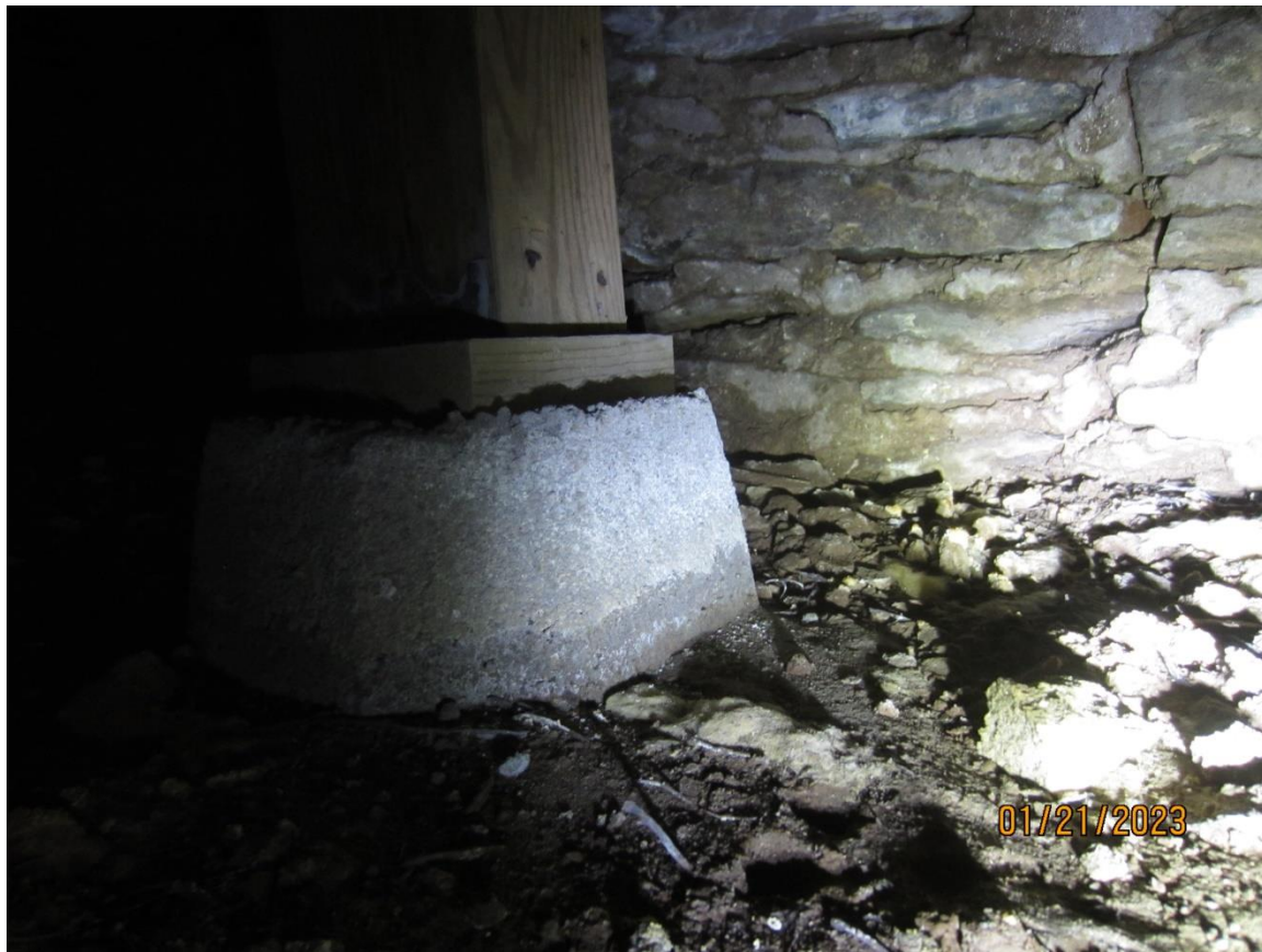
Pic 21 – Moisture at pier block and stacked shale foundation wall at Gridline 2.
