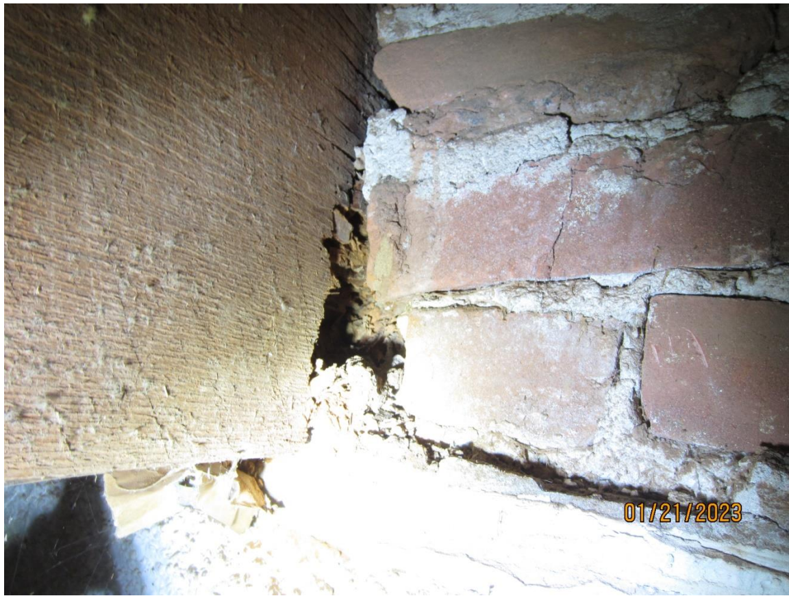
Pic 11 – Dry rot at embedded 2"x11.25" attic floor joists
