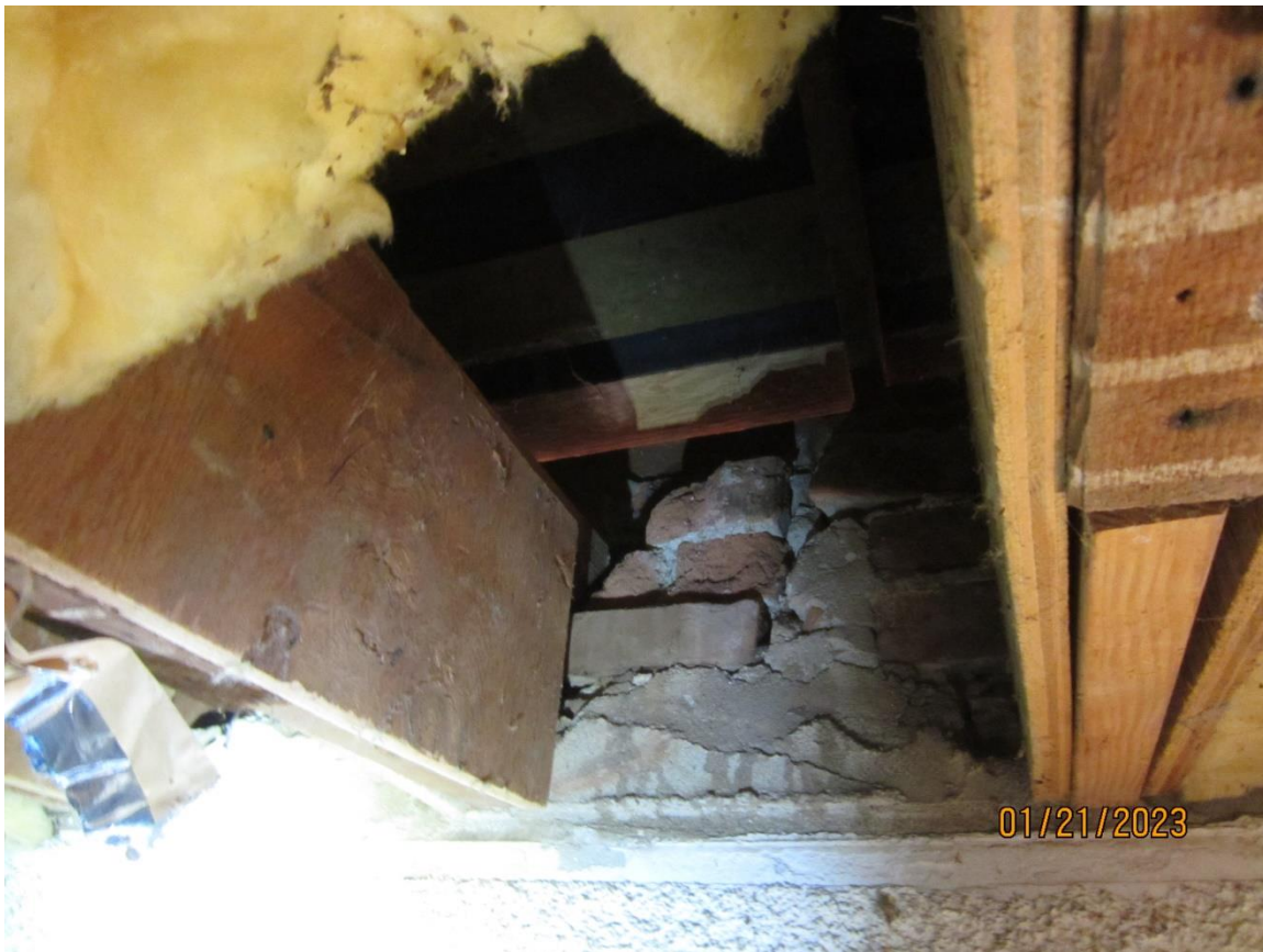
Pic 14 – Weak mortar and loose bricks at attic ceiling joist repair locations.
