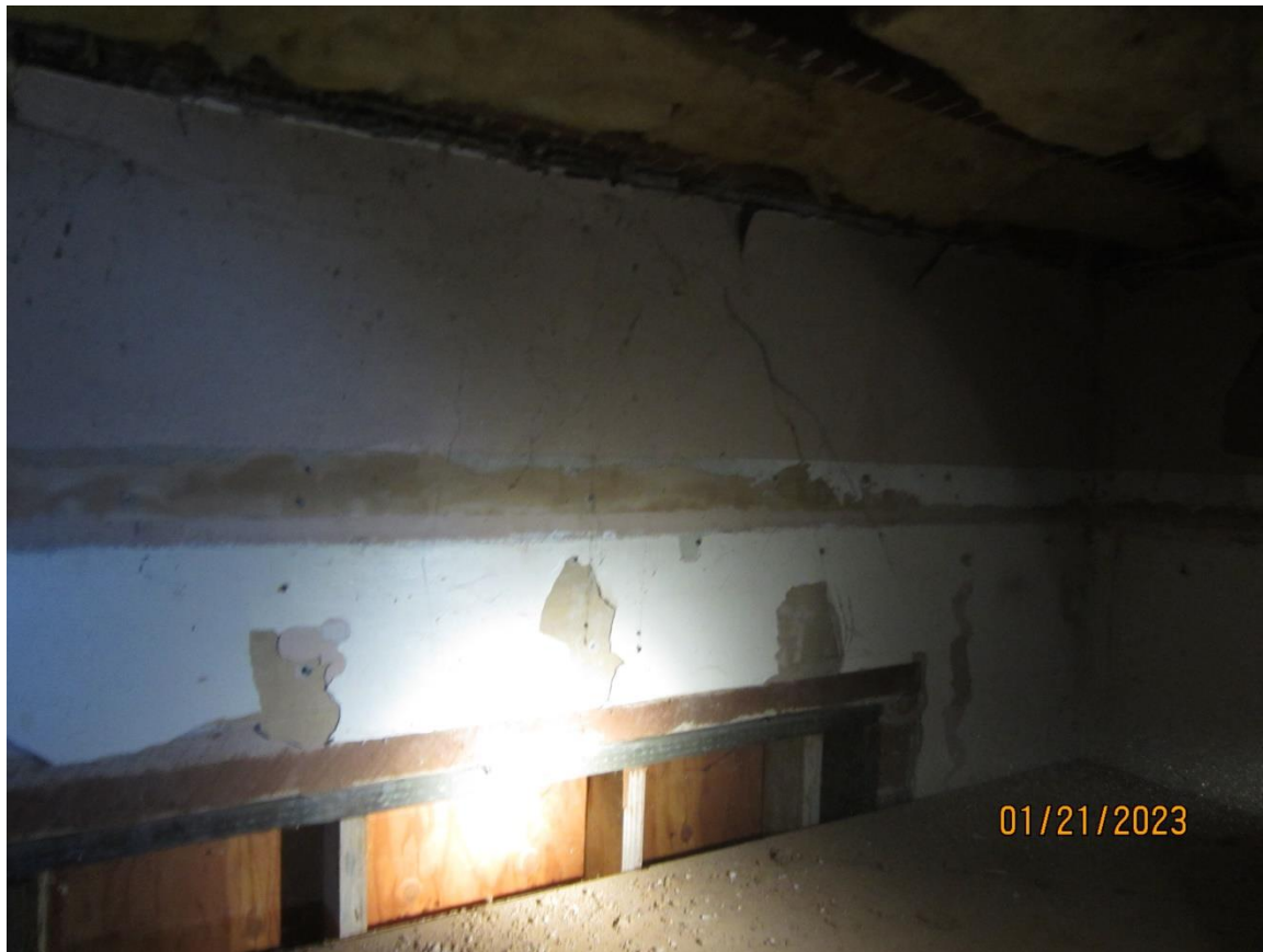
Pic 9 – Added hard lid ceiling below attic ceiling joists at northwest corner of URM building.
