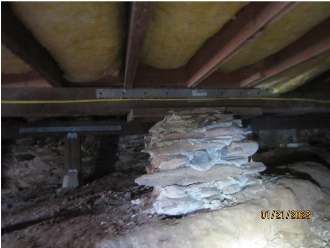
Pic 26 - Beam splice over shim at built-up shale pier
