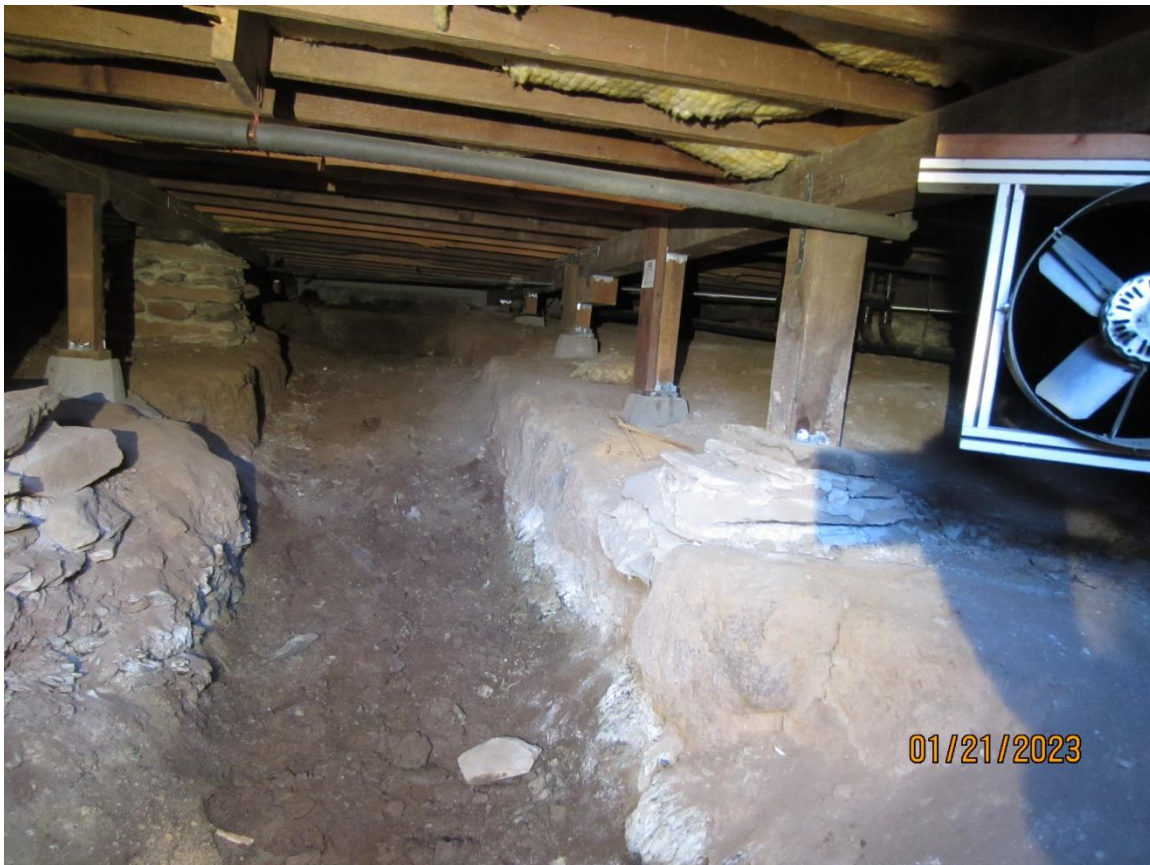
Pic 20 – Drainage trench sloping from east to west toward crawl space access door.
