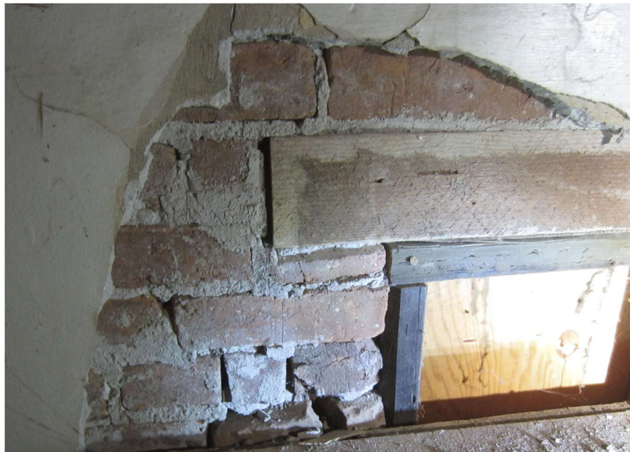
Figure 9 – Moisture affecting plaster and mortar
