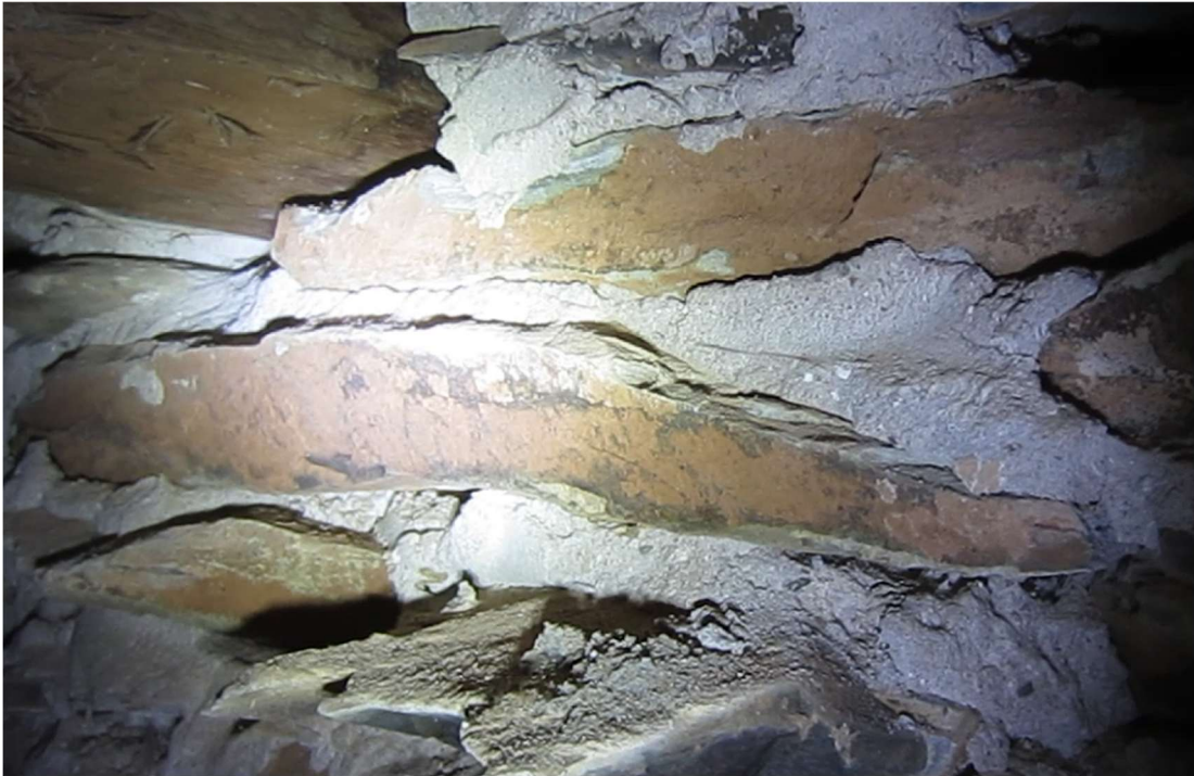
Figure 12 – Foundation Stacked Stone - Moisture affected mortar strength
