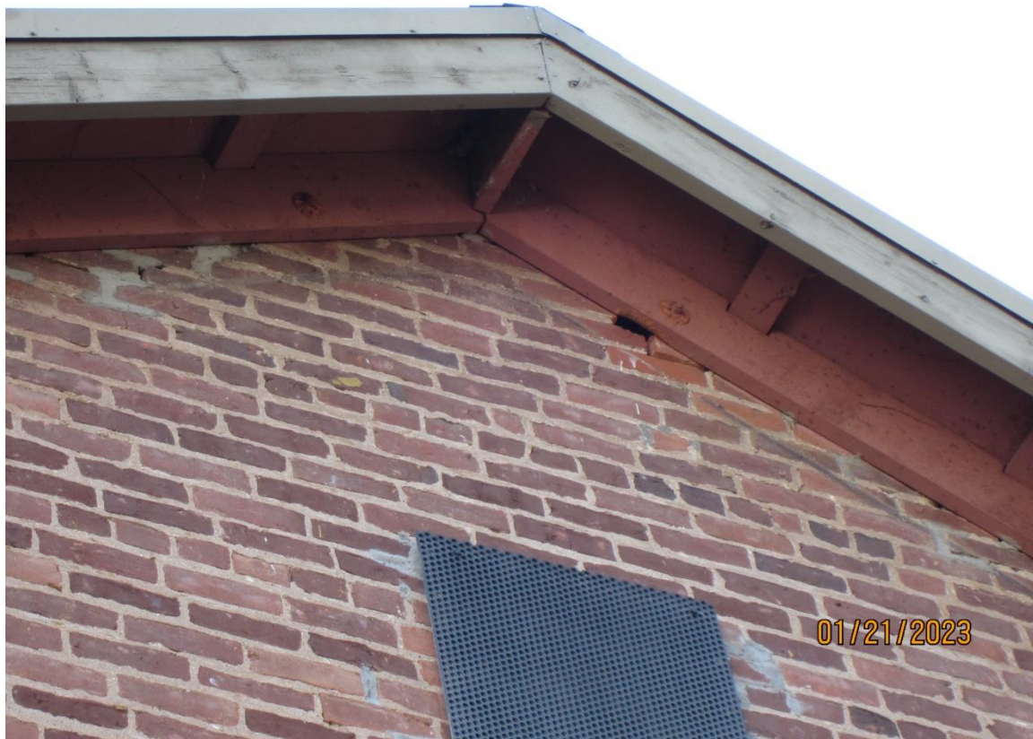
Pic 18 – Loose and missing bricks at west wall gable
