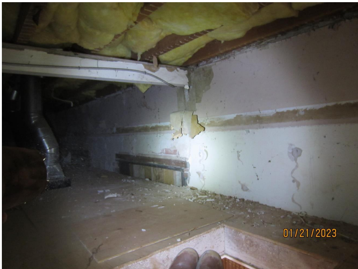
Pic 8- Hard lid ceiling with ½" plywood at west wall added per 1991 structural plans w/ attic floor joists above.
