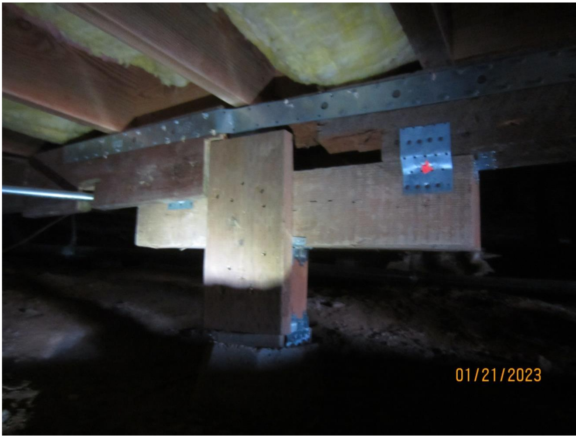
Pic 27 – Beam splice and dry rot repair over pier block (teter-totter method)
