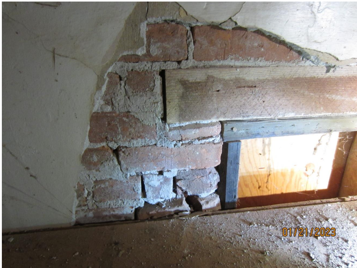
Pic 2- Brick and mortar at wall openings at West Wall at 1991 Hard Lid Ceiling with plywood diaphragm+
