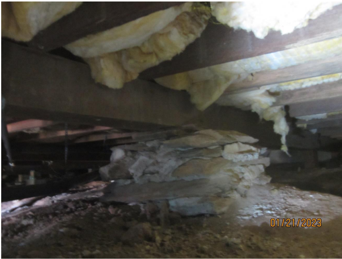
Pic 25 - Floor beam supported on stacked shale pier
