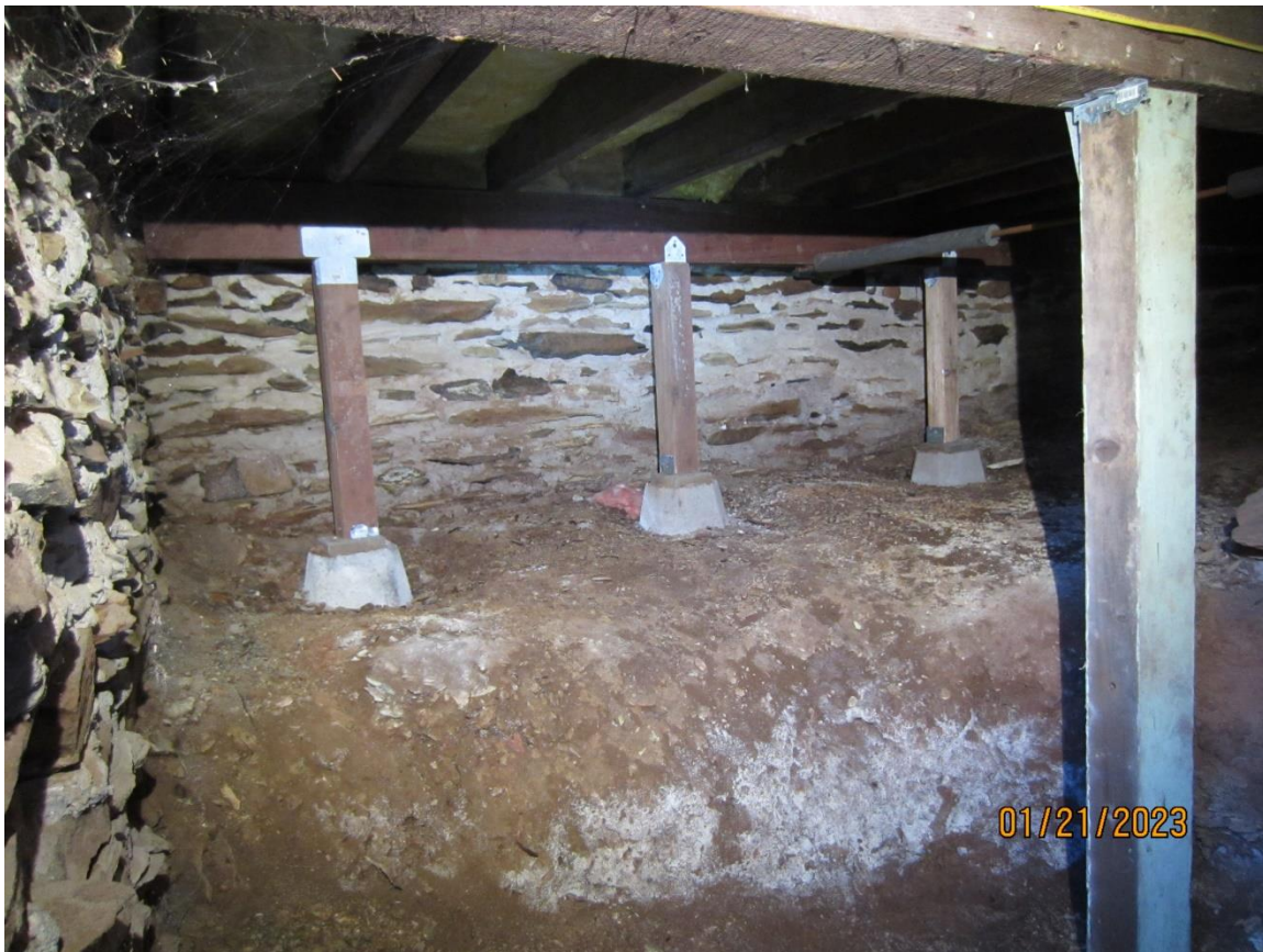
Pic 24 – Stacked shale foundation wall at southwest corner of crawl space.
