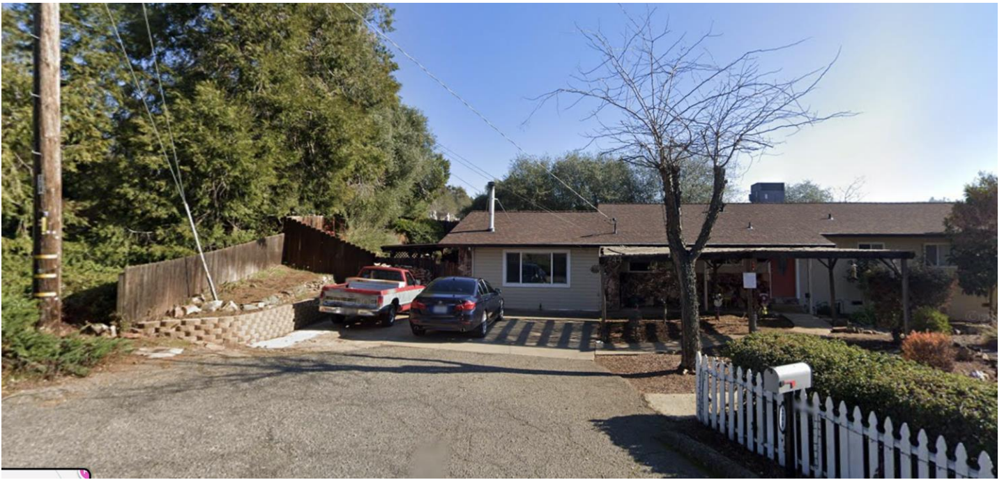
FIGURE 2 – STREET VIEW- 244 Oak Court
