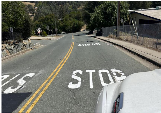
Finished Pavement Markings around Amador High School
