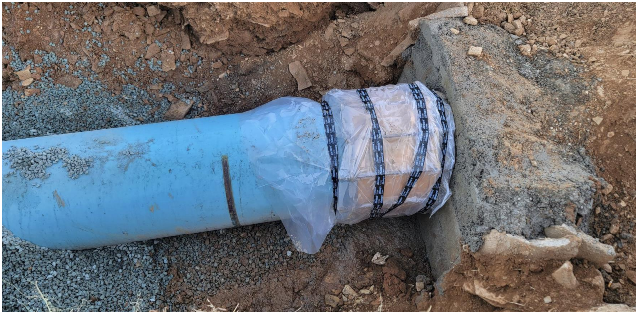
Top Joint repaired
