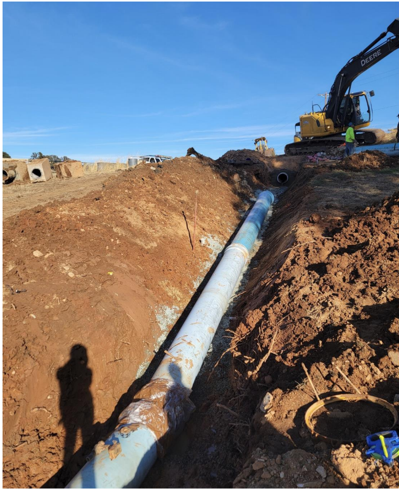
Pipeline repair, full extent
