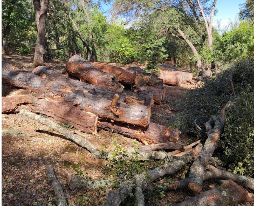
Tree dropped to ground and partially bucked up
