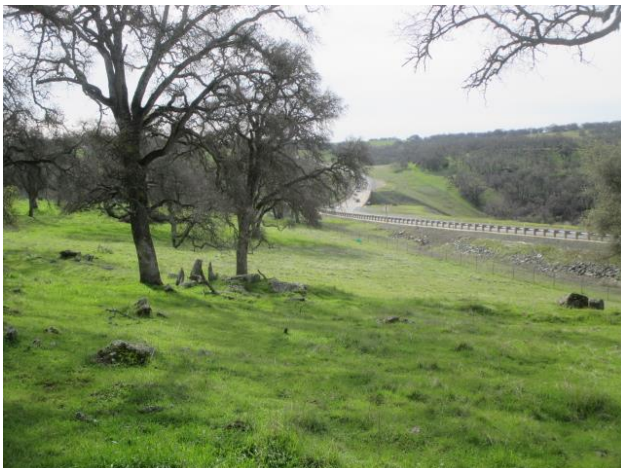
Hwy 49 Guardrail at Westerly Boundary of Site
