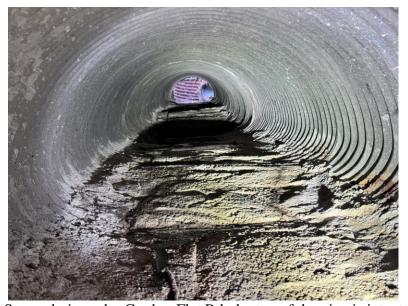
Storm drain under Gopher Flat Rd. the top of the pipe is intact.
