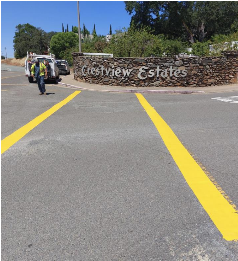
Crestview Estates Crosswalks
